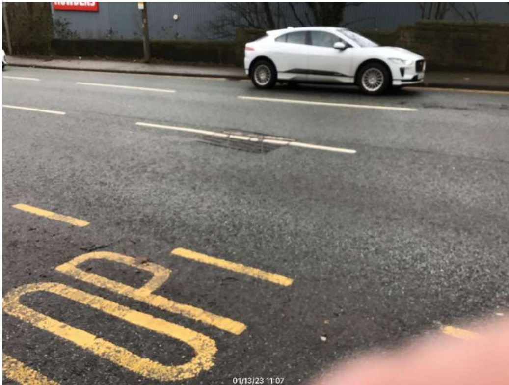
16) South of bridge, Northbound Lane 1: Cracks to surface course nest to gully
