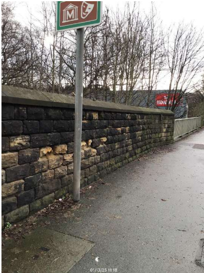
38) North of bridge, East footway wall: Existing condition
