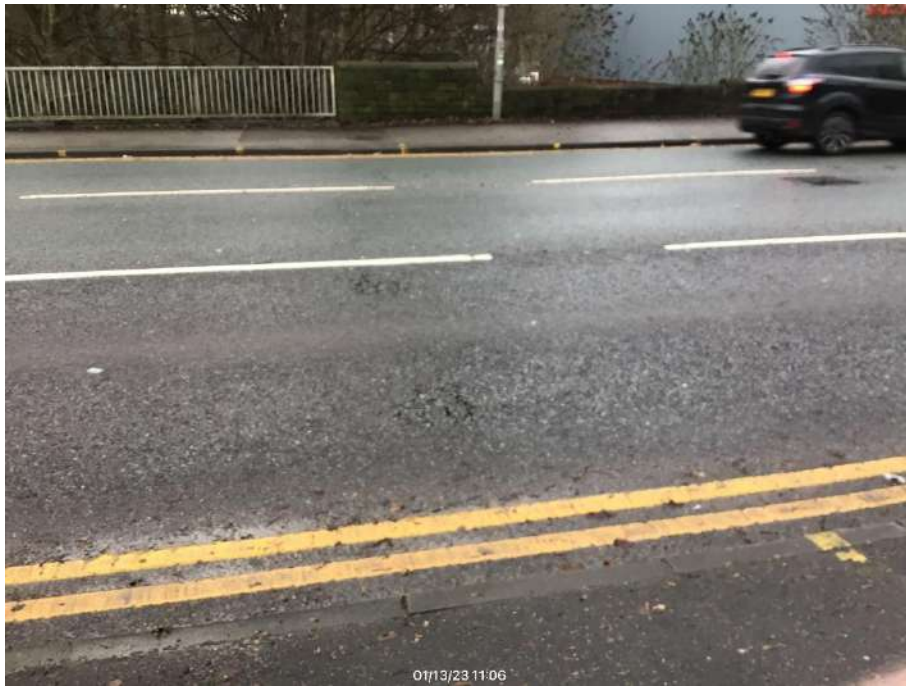
14) South of Bridge, Northbound: Blocked gully
