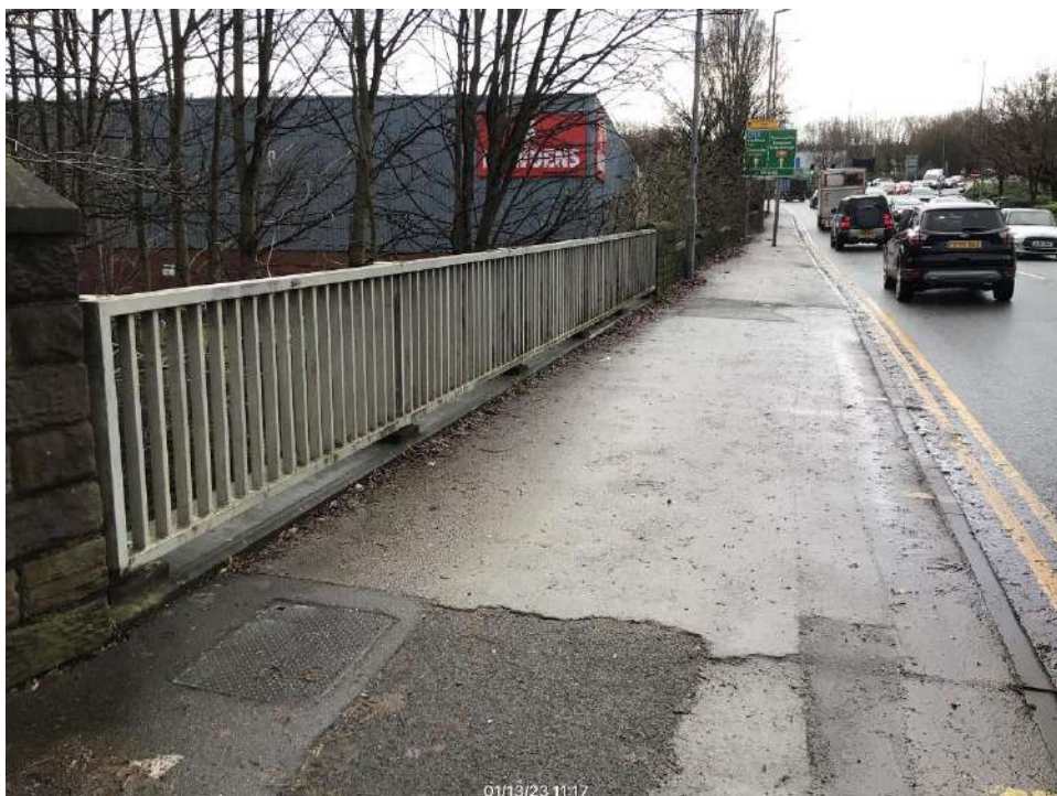
34) North of bridge, East footway: Existing footway tarmac/East Parapet
