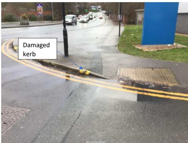
5) Northwest tie in: Damaged kerb/standing water to pedestrian crossing
