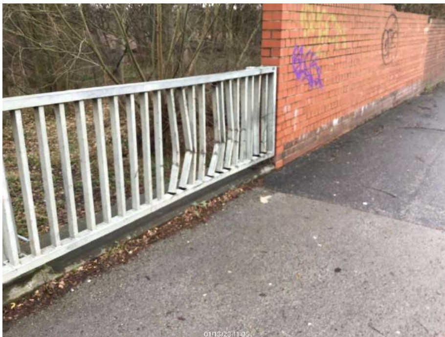
12) Damage to west bridge parapet
