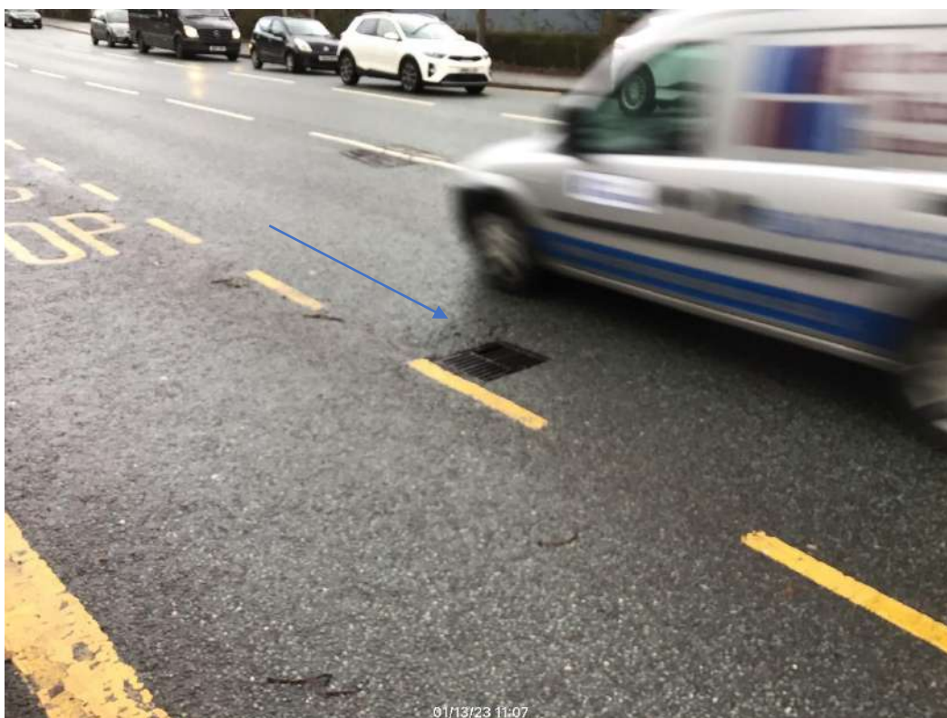
16) South of bridge, Northbound Lane 1: Cracks to surface course nest to gully
