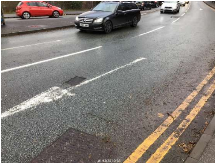
3) Lane 1 Northbound: low chamber/water valve
