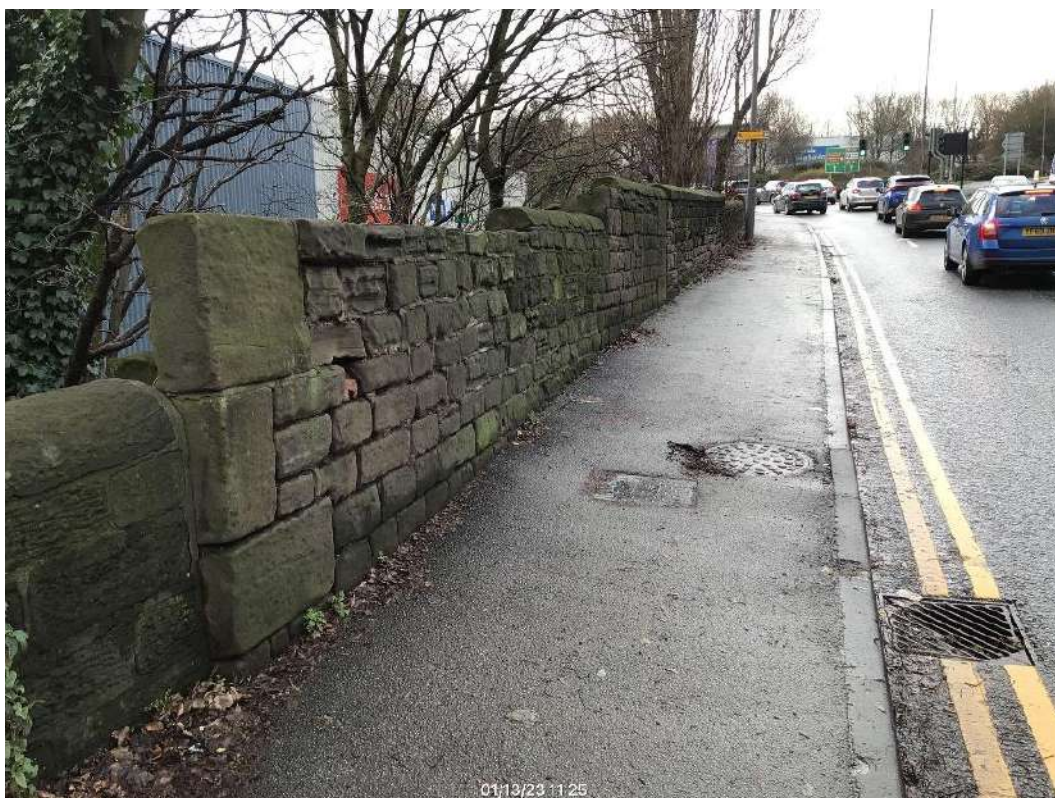
30) South of bridge, East footway wall: Existing wall condition
