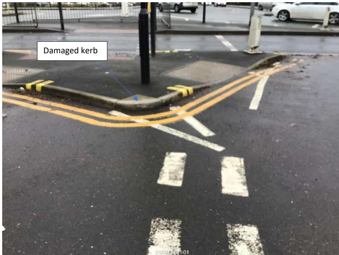
6) Northwest tie in: Damaged kerb
