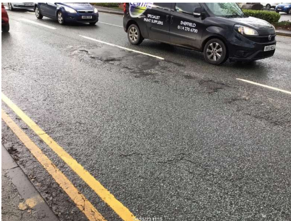
28) South of bridge, southbound: failed surfacing course
