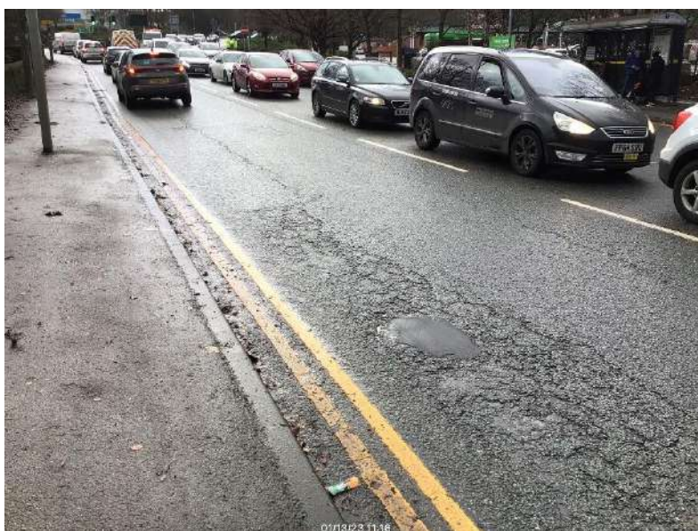
32) South of bridge, southbound: Failed/cracking to surfacing course
