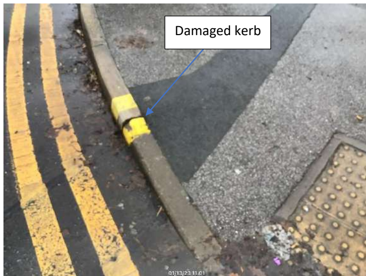
6) Northwest tie in: Damaged kerb
