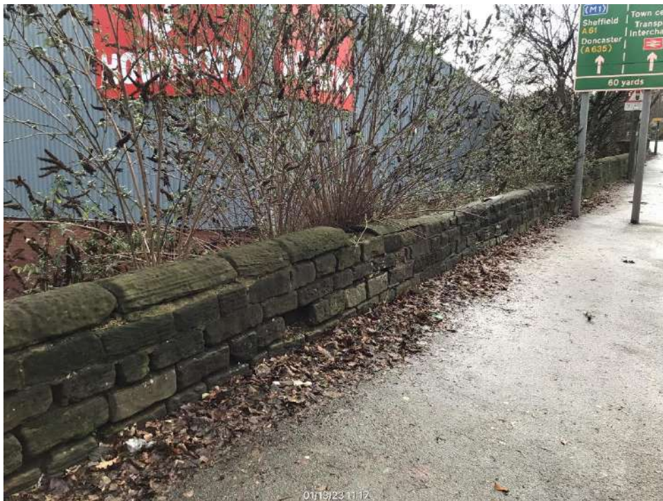
33) South of bridge, East footway: Existing wall condition
