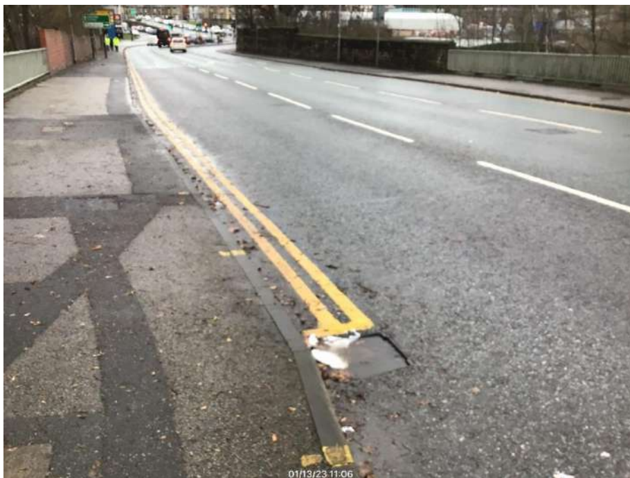
14) South of Bridge, Northbound: Blocked gully
