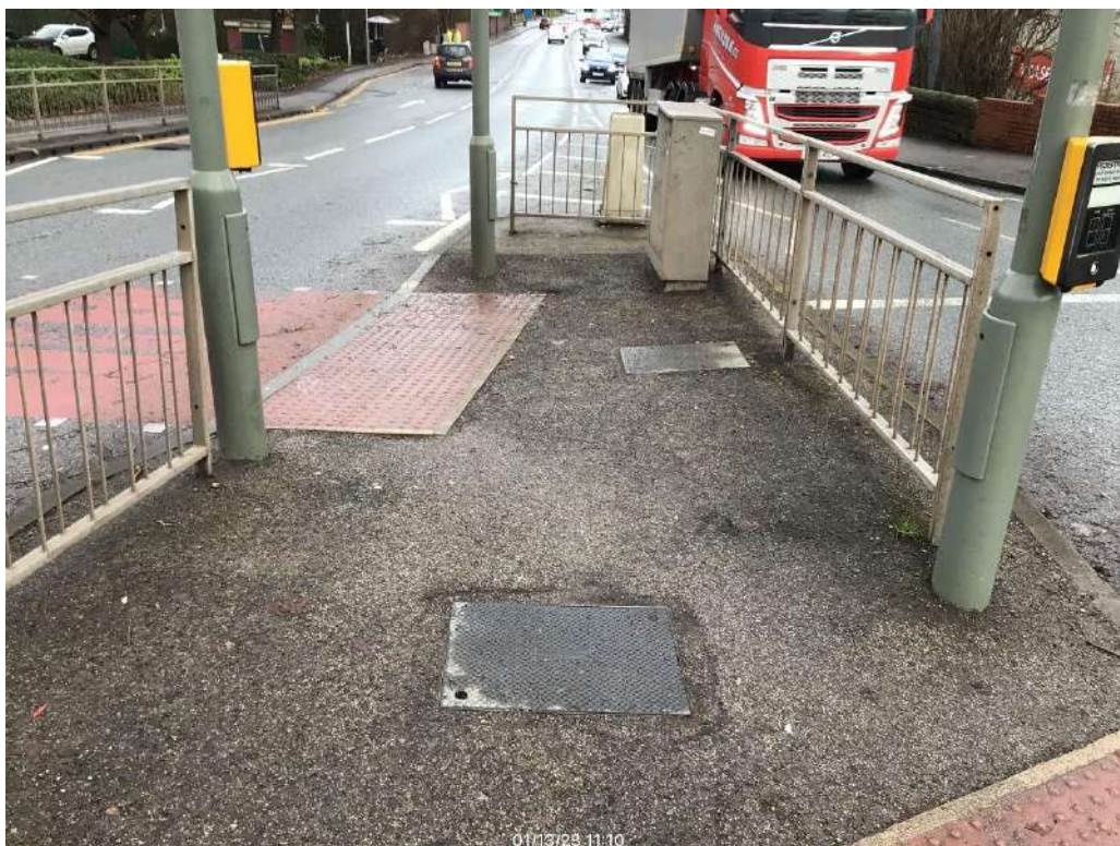
20) South tie in pedestrian crossing island: low chamber with sunk tarmac surround
