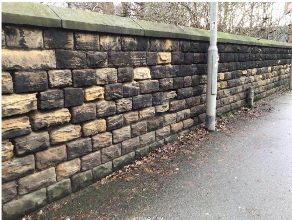
39) North of bridge, East footway wall: Existing condition
