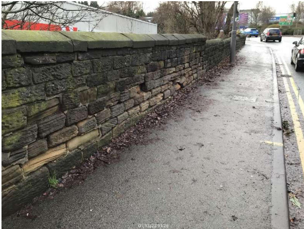
26) South of bridge, East footway wall: Existing condition
