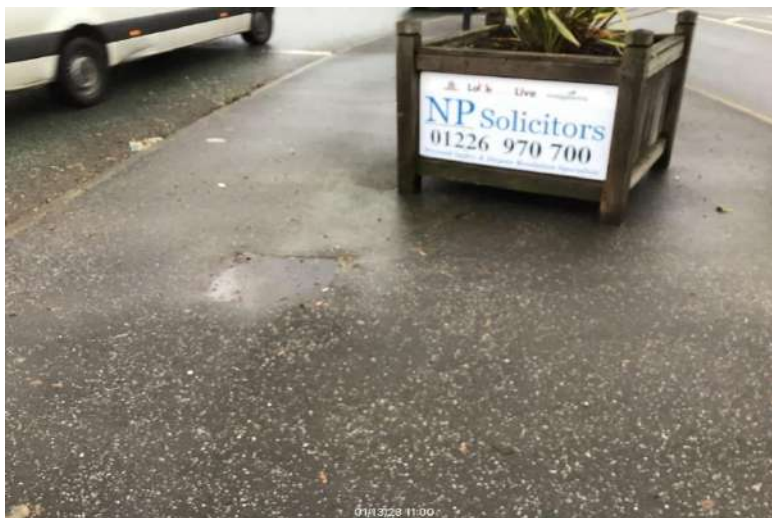
5) Northwest tie in: Damaged kerb/standing water to pedestrian crossing
