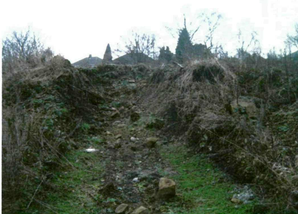
Photograph number 7 showing the excavations in the tip and illustrating the type of material tipped by the Council which is rubble, brick, concrete and sandstone kerbs and setts.
