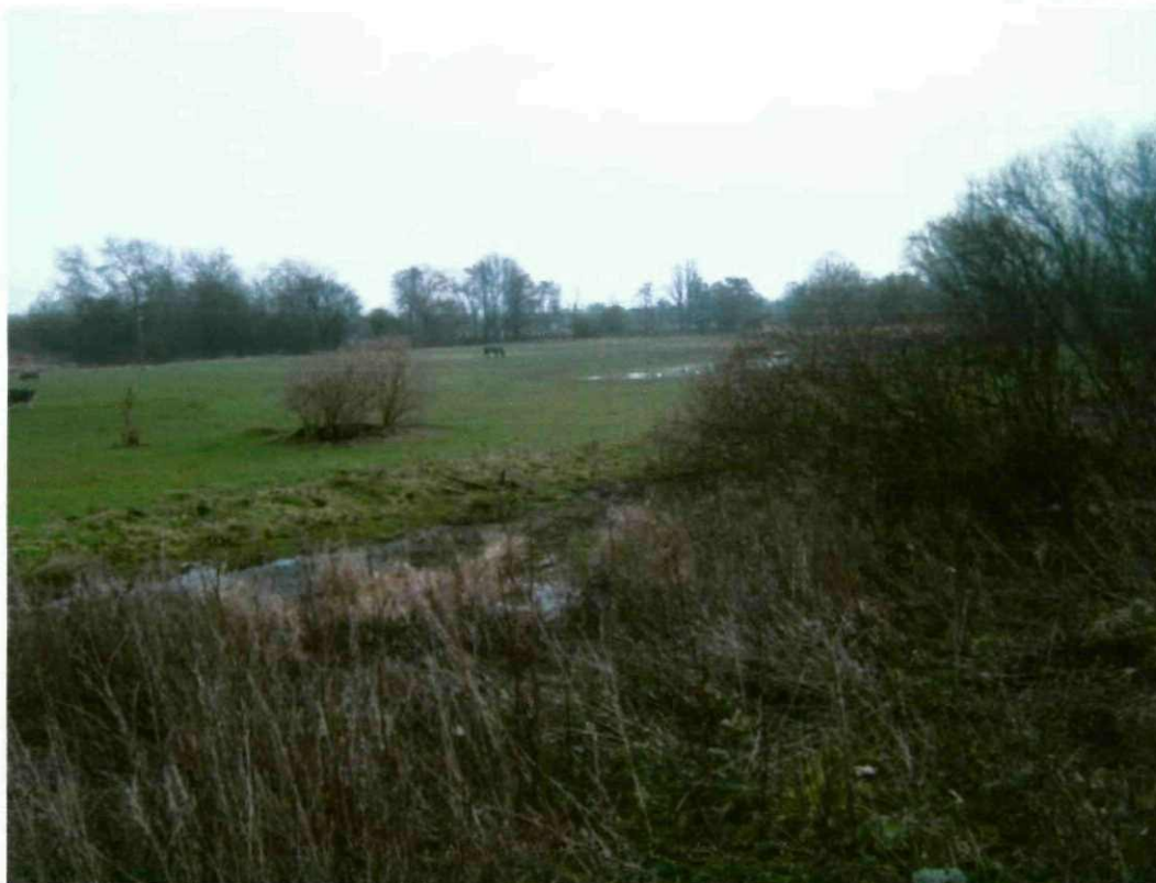
Photograph number 29 showing the stream on the side of the tip and flood area widened out at the field side and the base of the tip.
