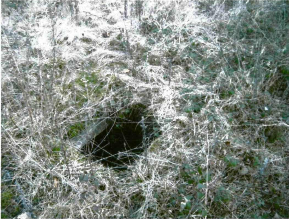
Photograph number 27 showing an old manhole which will be inspected and any pipe renewed if run off from the site.
