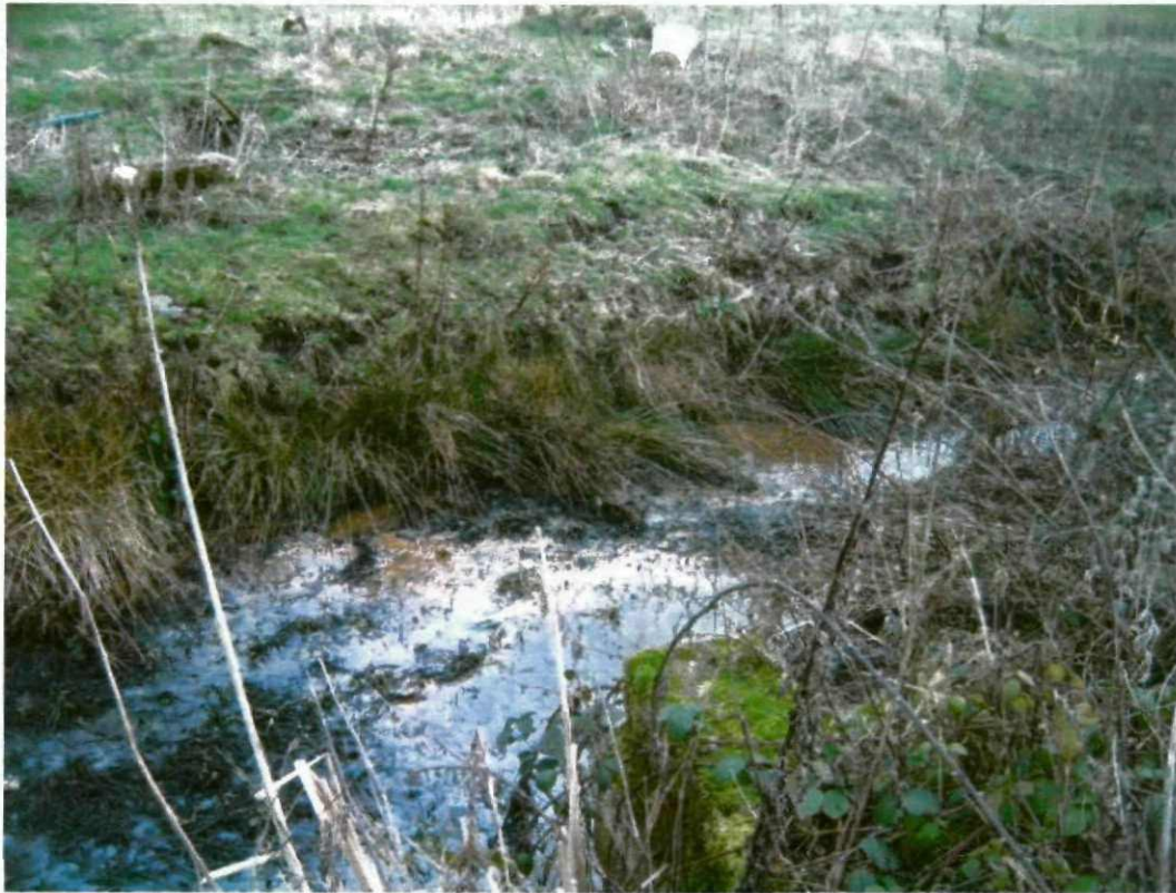
Photograph number 17 showing the stream with ochre water in it and heavily choked with vegetation, which will be cleaned out.
