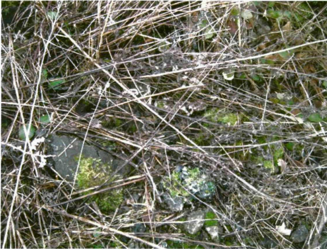
Photograph number 33 showing a close up of the rubble and tarmac on the site from the Council's highway works.
