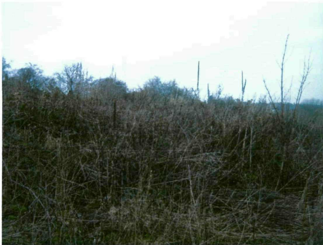
Photograph number 34 showing the slope of the tip from the stream looking north.
