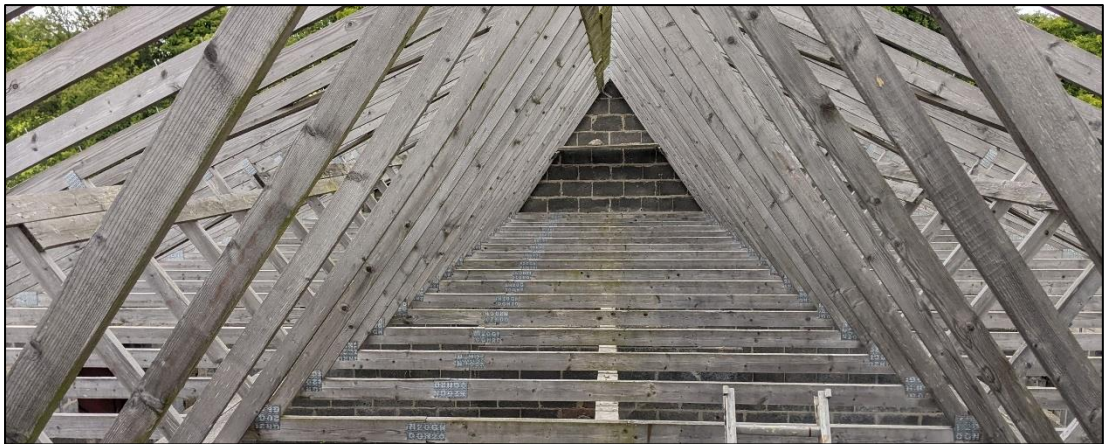
Plate 4. Prefabricated trusses in roof of former stables
