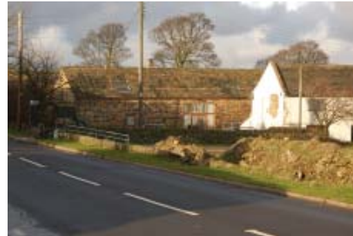
Approach to the site
