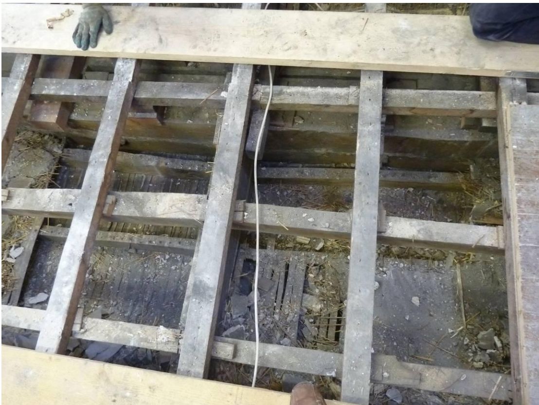
6 Photograph of the structure from above. The lime mortar and straw pugging has been partly removed to expose the lath and plaster. The re-used riven or rough-hewn floor joists are apparent at the bottom of the photograph. The one beneath the joiner's knee is modern sawn softwood. The repair to the principal beam is apparent (see below)
