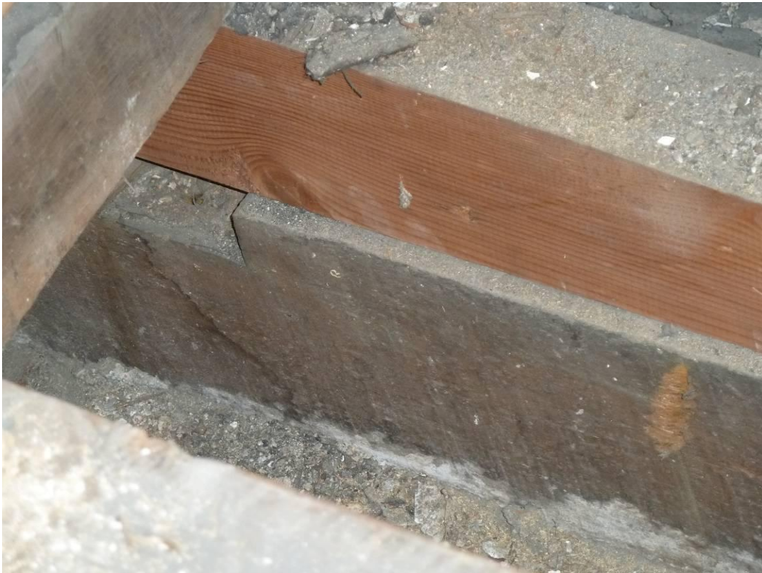
7 Mortise in secondary beam – former housing of floor joist – and modern levelling member.
