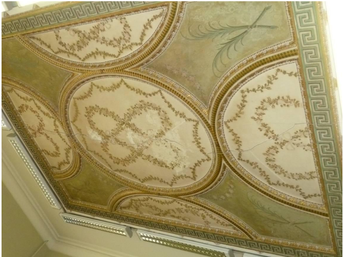
11 Ceiling of more westerly room: NB Painted decoration, moulded and gilded radius work within decorated key pattern border. There is a cornice at the wall to ceiling junction- installed after the ceiling was lowered in 1950.
