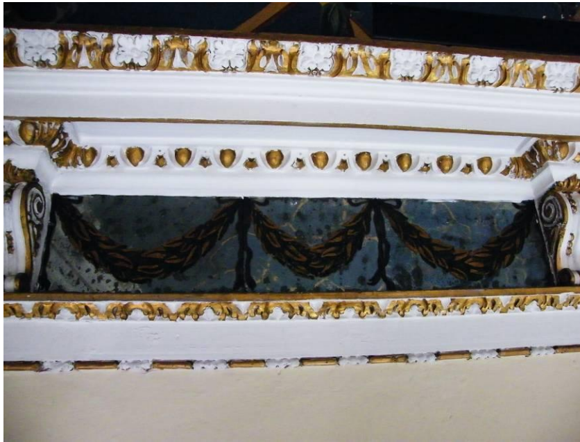
23 Existing cornice and frieze in the Aviary Room of the South Palladian Wing
