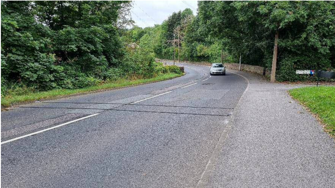
Photo 1: Keresforth Road (B6099)
