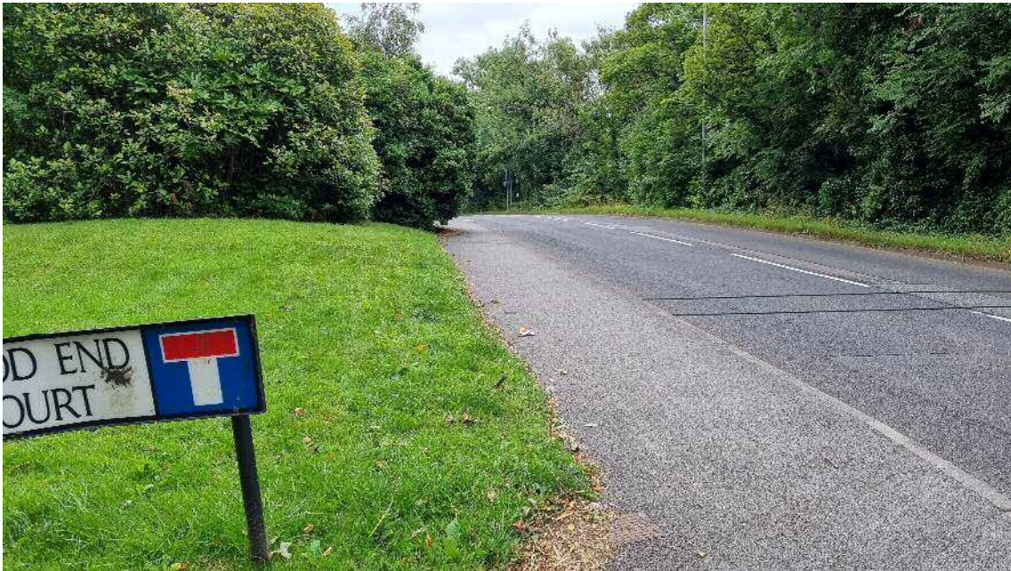
Photo 3: Footway on Keresforth Road
