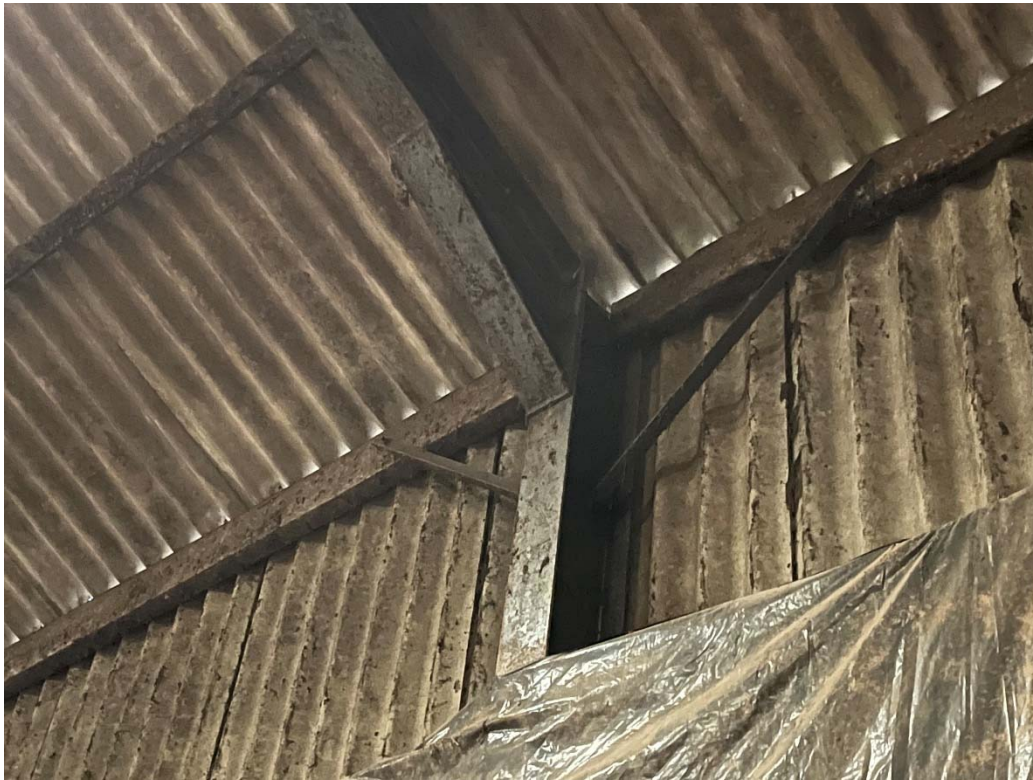
Photograph 5 Building 14 Typical Cladding
