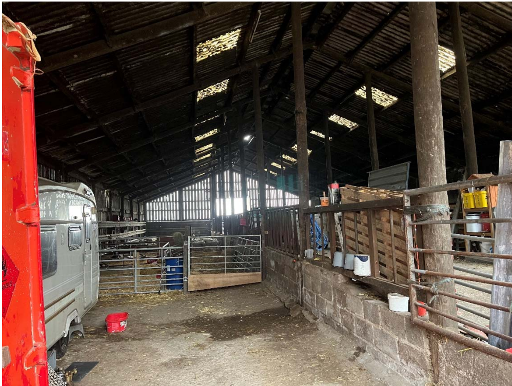
Photograph 1 Building 8 Internal View
