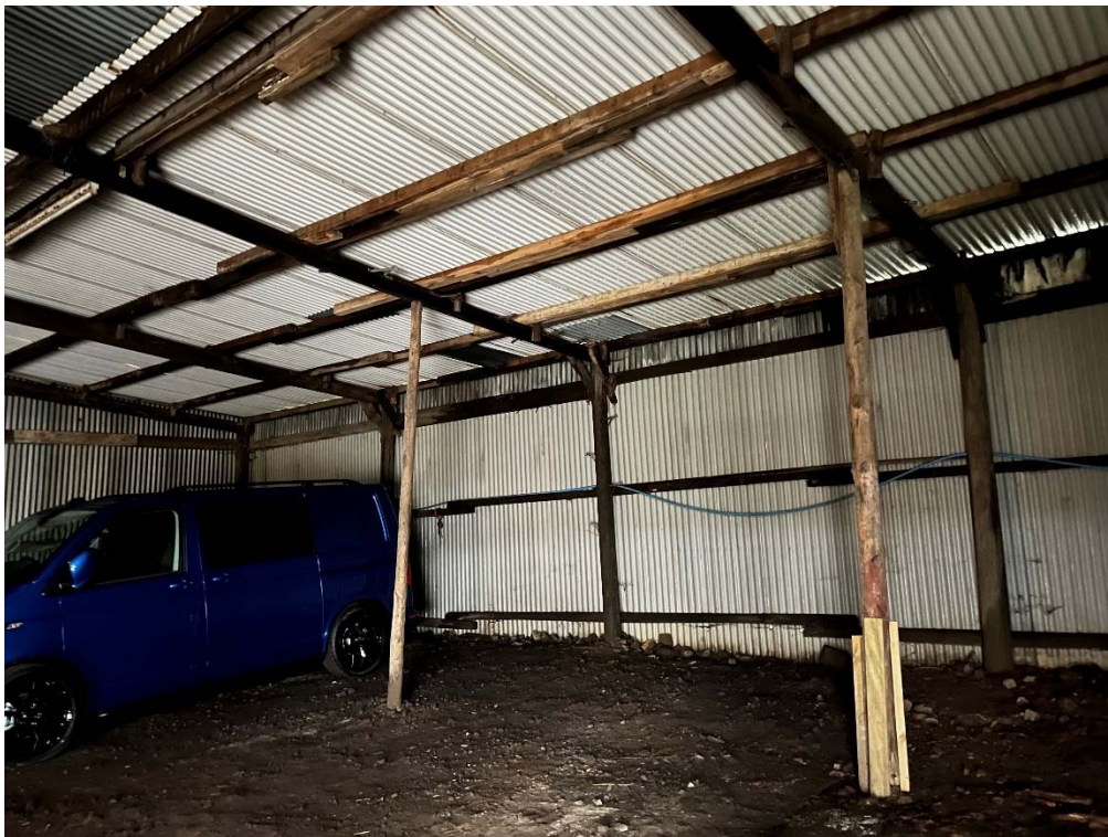
Photograph 8 Building 19 Typical Cladding
