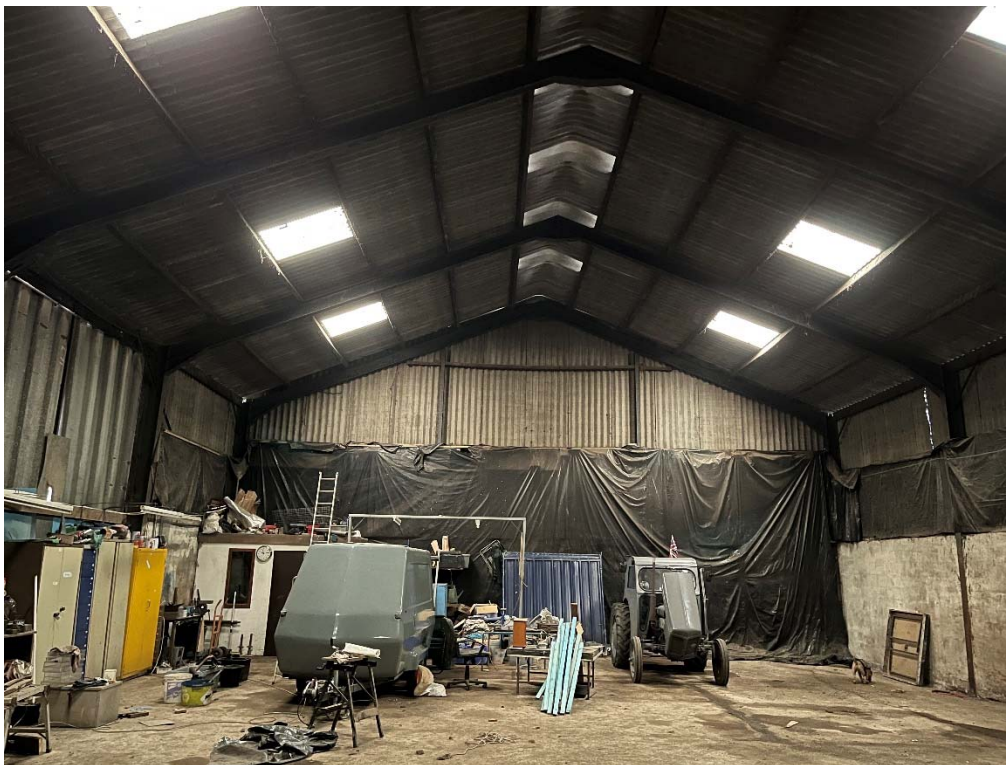
Photograph 4 Building 14 Internal View
