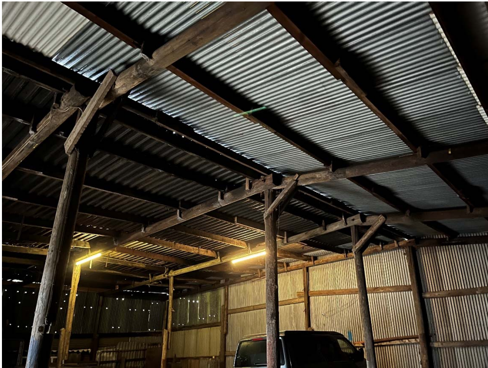
Photograph 7 Building 19 Internal View
