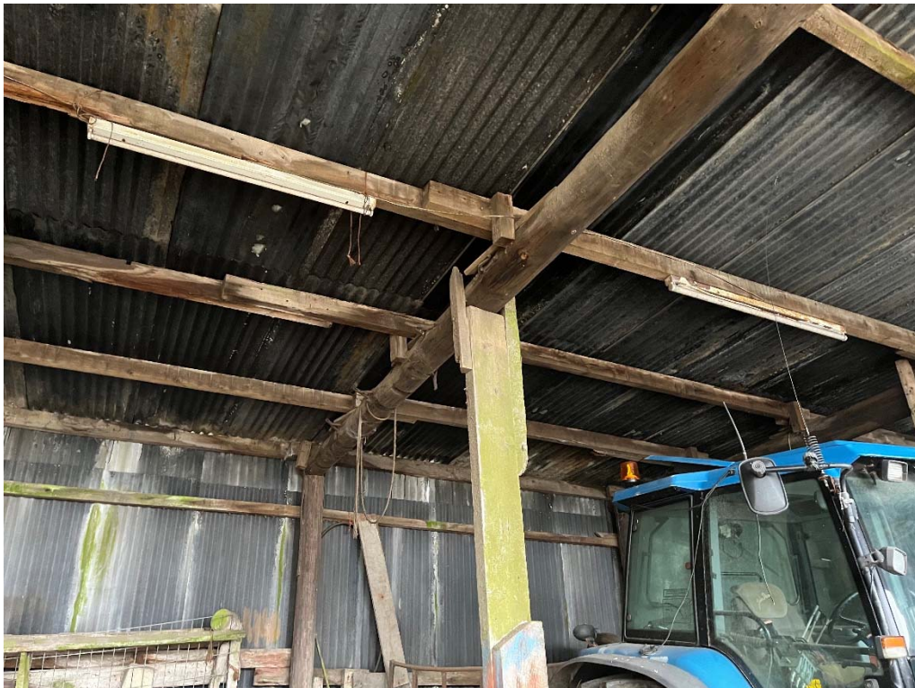
Photograph 11 Building 20 Internal Cladding
