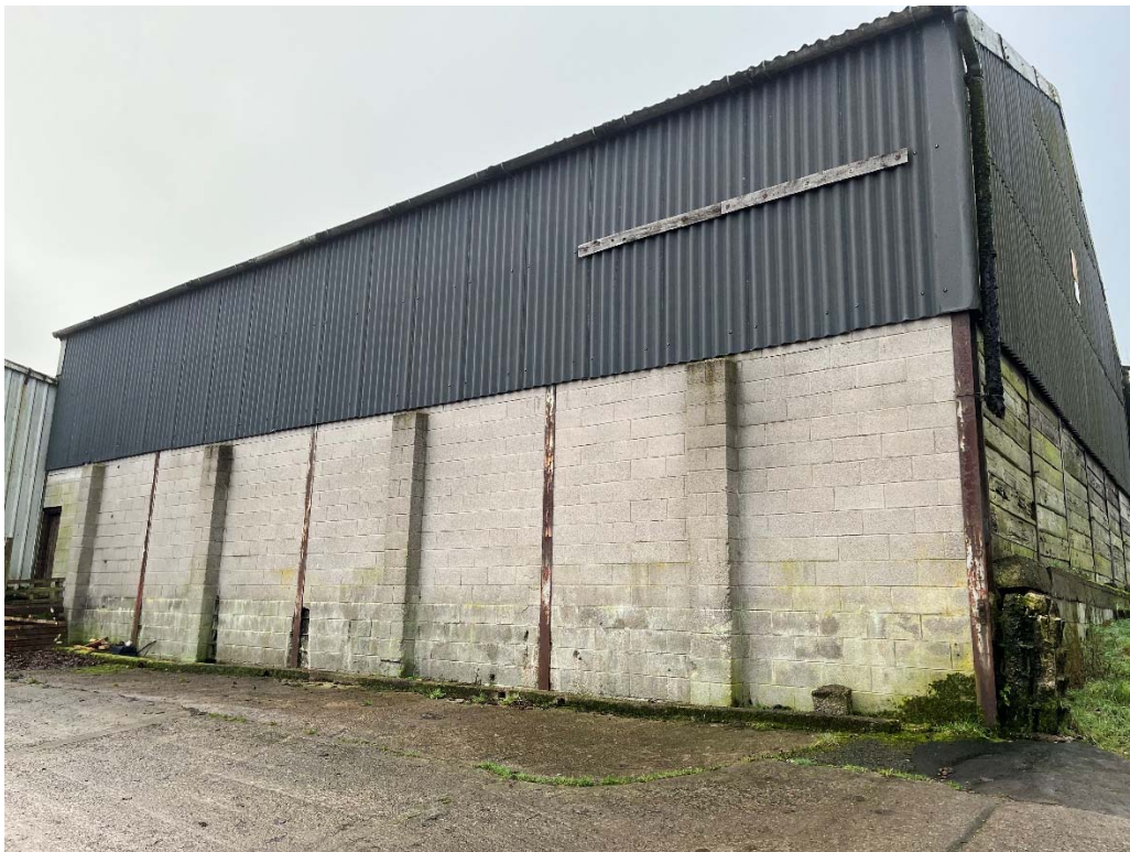
Photograph 6 Building 14 Western Elevation Retaining Wall
