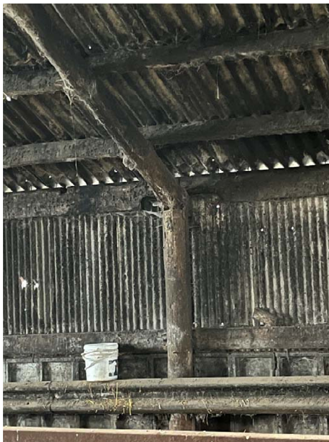
Photograph 2 Building 8 Typical Cladding
