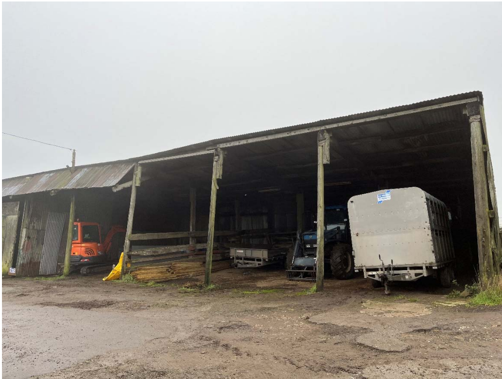
Photograph 10 Building 20 Front Elevation
