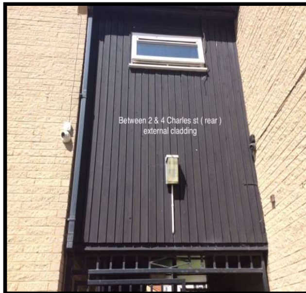
No. 2 – 4 Charles Street - Rear Elevation
