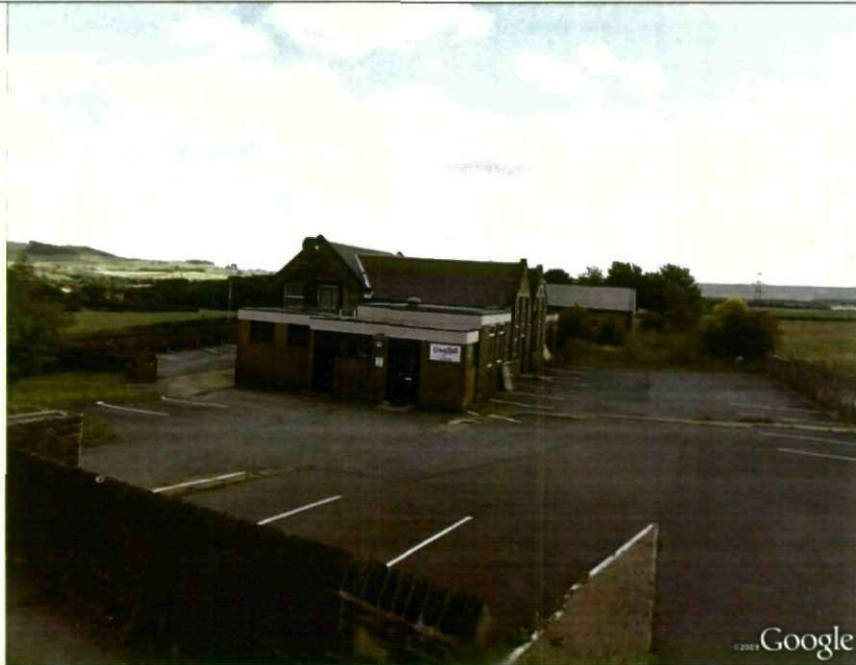
Figure 2: Existing Building Viewed South East
