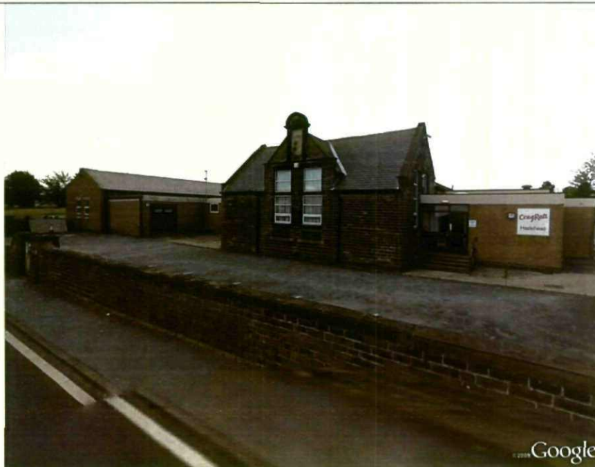
Figure 3: Existing Building Viewed South West
