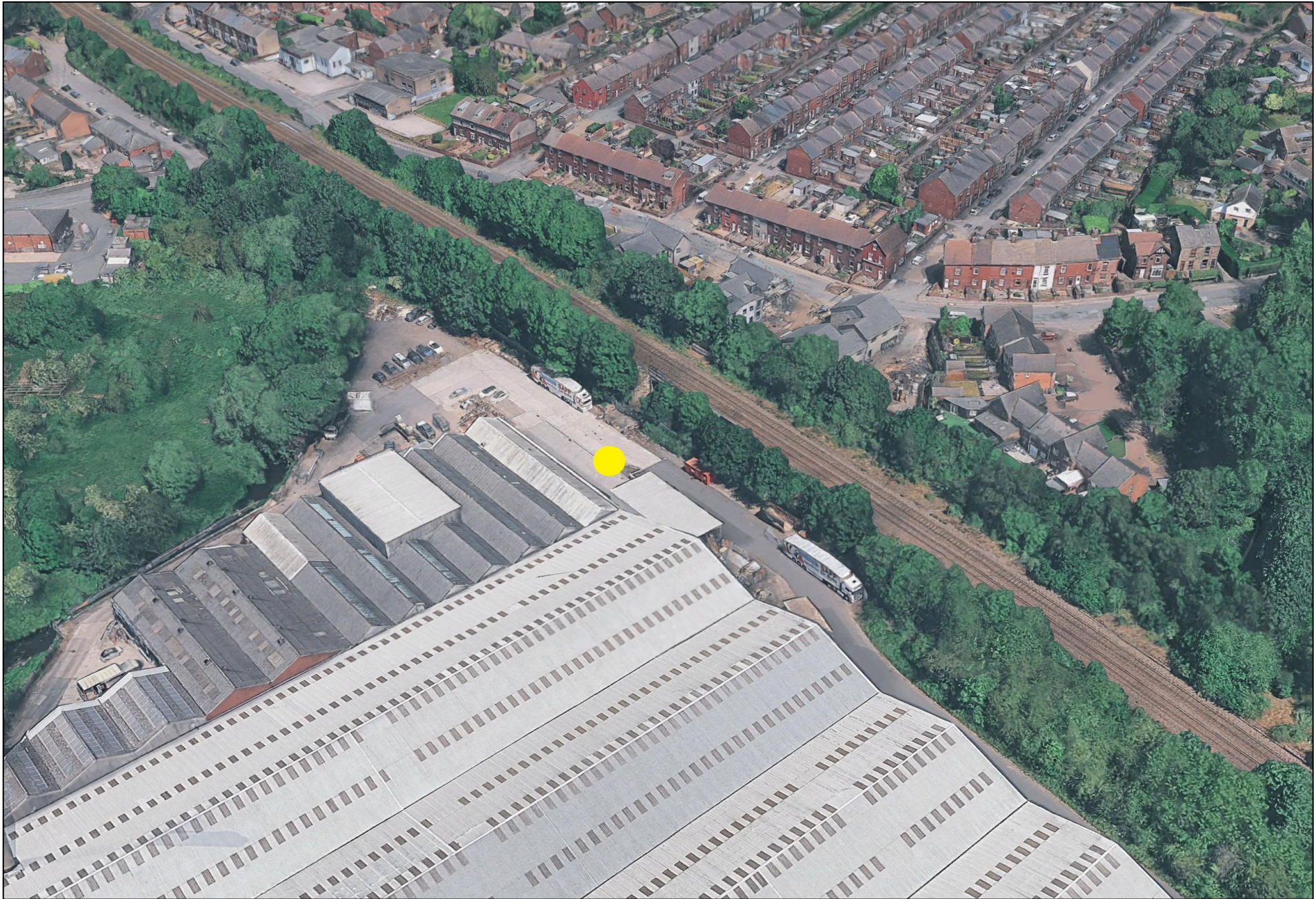
FIG 1: DARTON BUSINESS PARK, BARNSELY (showing monitoring location)
