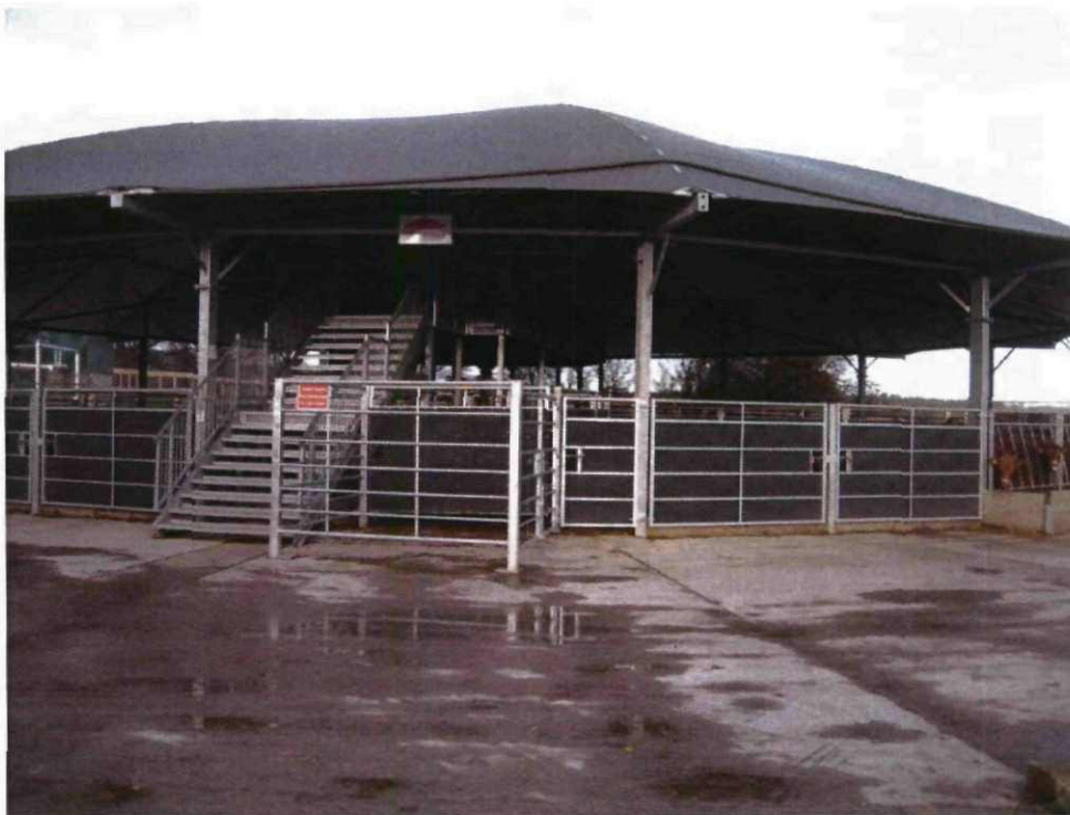
14. The roundhouse. A state-of-the-art stock building with high level gantry for public viewing.
