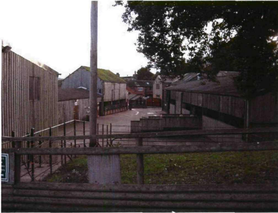
13. Existing animal buildings at the centre of the site which need to be replaced as a result of the Griffin Report.
