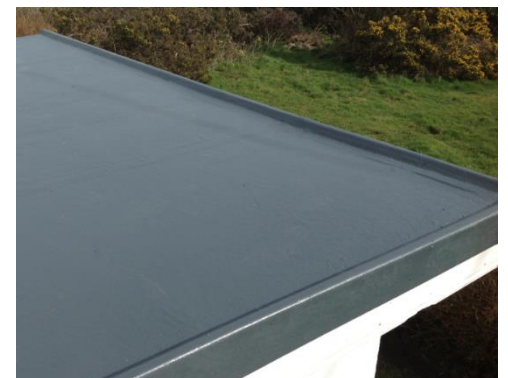
4. GRP roof finish
