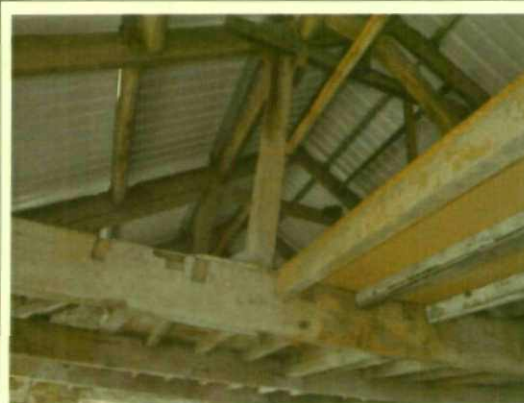
8 View within existing building – roof trusses
