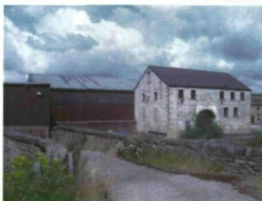
2 View of over the bridge to the East of the site looking at the existing void between the existing buildings (proposed site)
