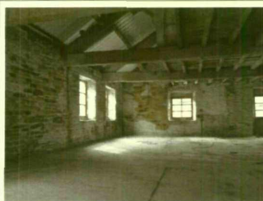
7 View within existing building – roof trusses
