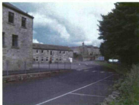
5 View from Eastern boundary (existing adjoining stone building to left) looking North West towards dwelling (Bullhouse Mill House)
