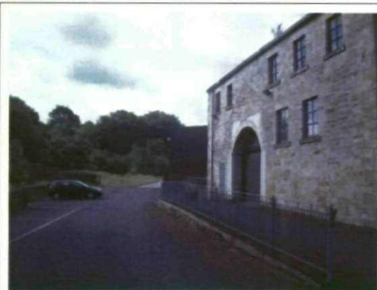
1 View of existing stone building (right) with proposed infill building in the distance
