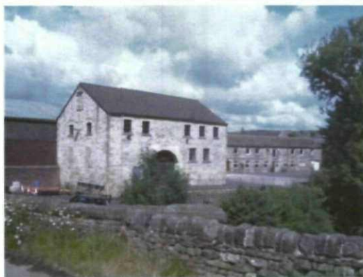
6 View from bridge looking West
