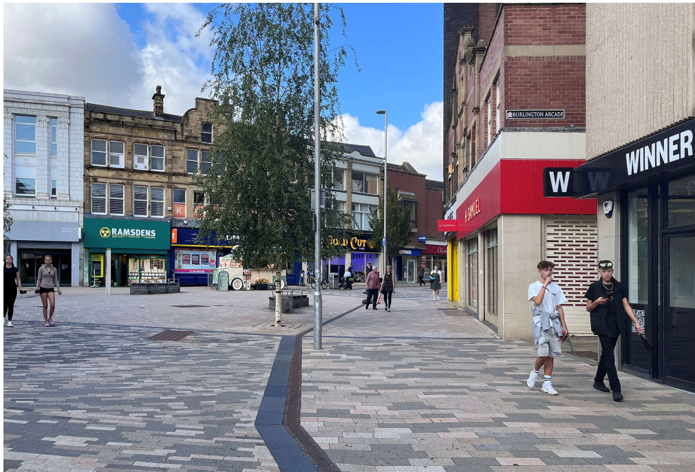
Existing Street View
