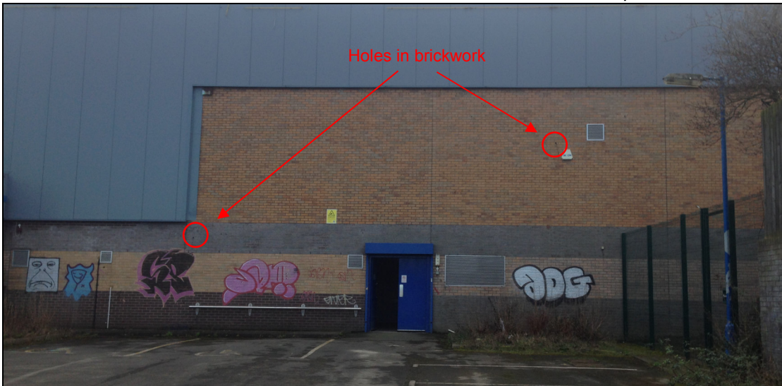
North-west elevation of building B1 showing potential access points
