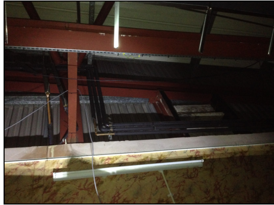
Metal construction of roof space
