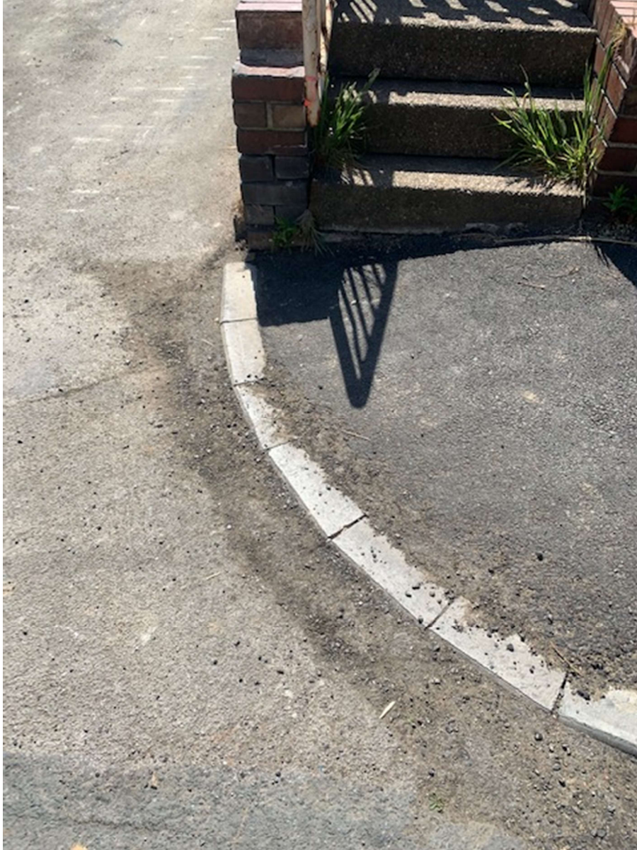
Site entrance northern radi
