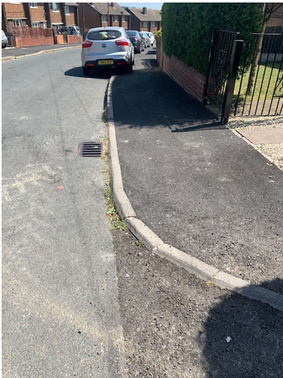
Site entrance looking south down Heysham Green
