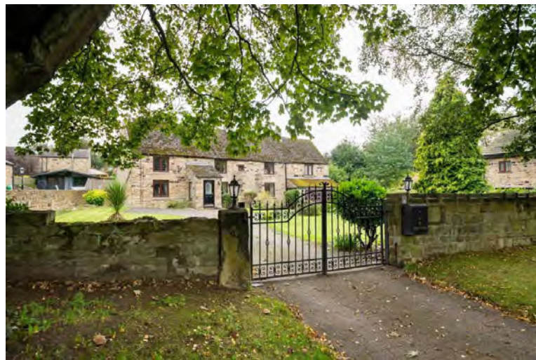
View Of Hirst Cottage From Chapel Lane
