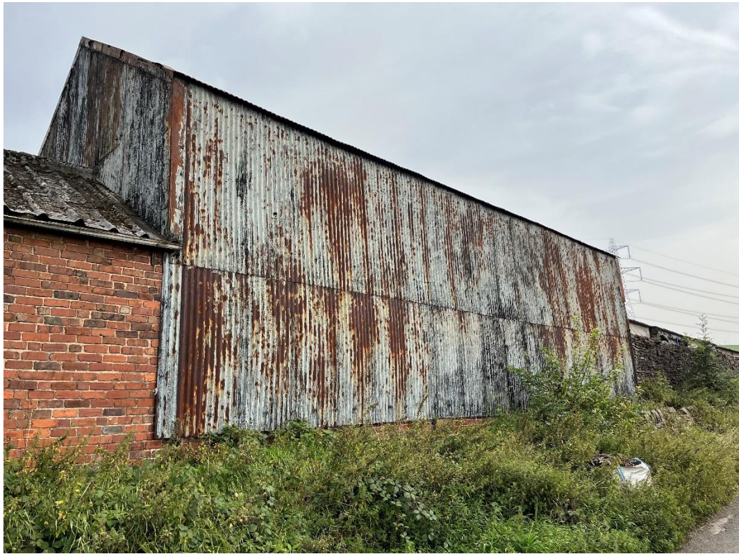
Photo P5 – The Old Cow Shed, Hunshelf Road Elevation
