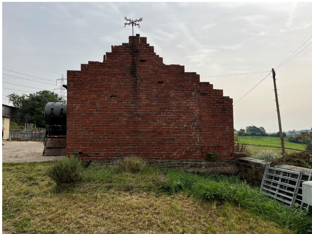
Photo P3 – Pony Stable Gable End
