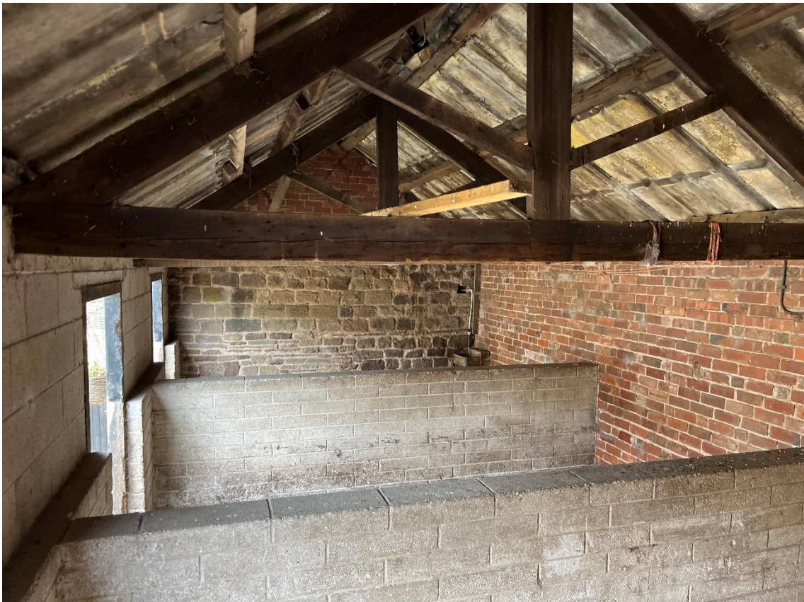
Photo P4 – Gable Separating Cow Shed/Stables and Roof Timbers
