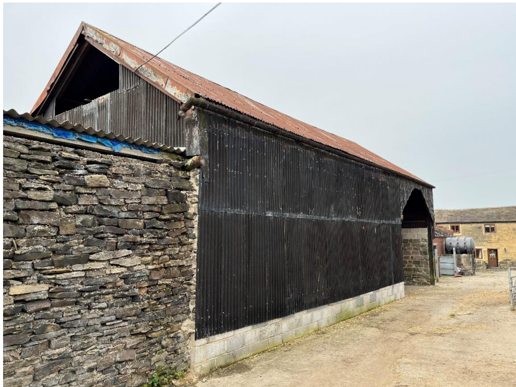
Photo P8 – The Old Cow Shed, Adjoining Wall to Storage Barn
