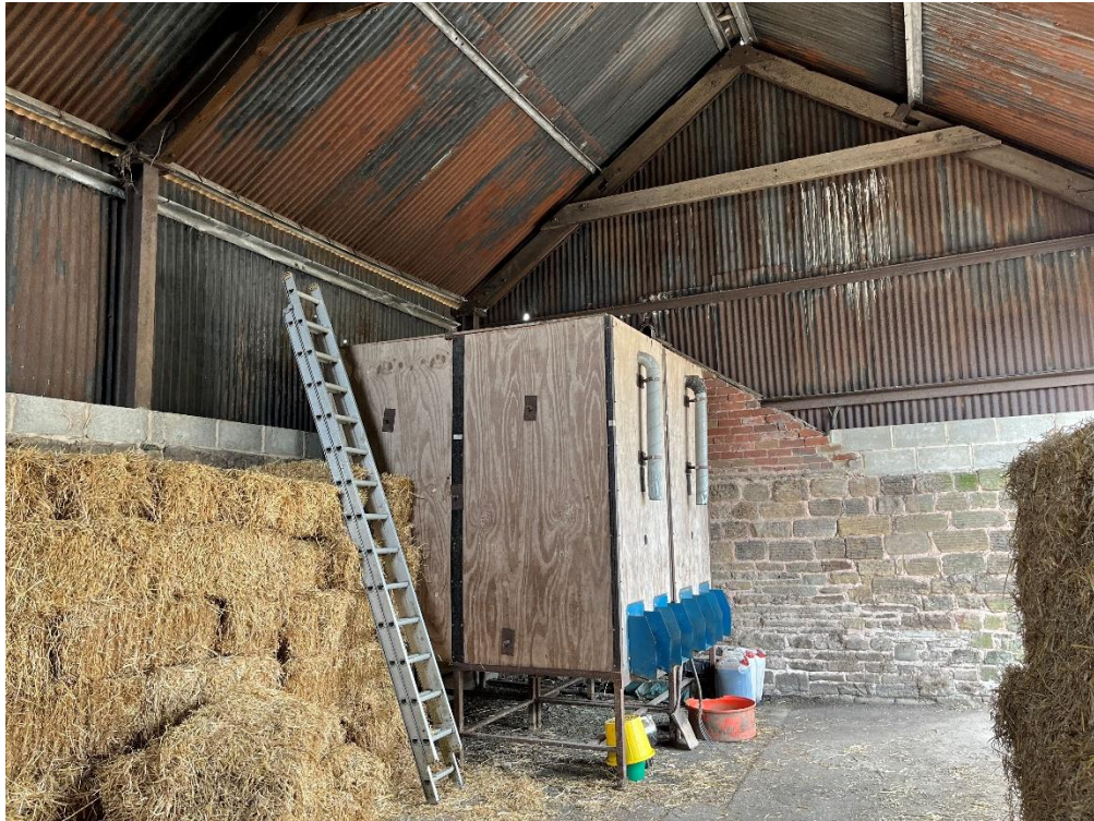
Photo P7 – The Old Cow Shed Adjoining Gable to Stables
