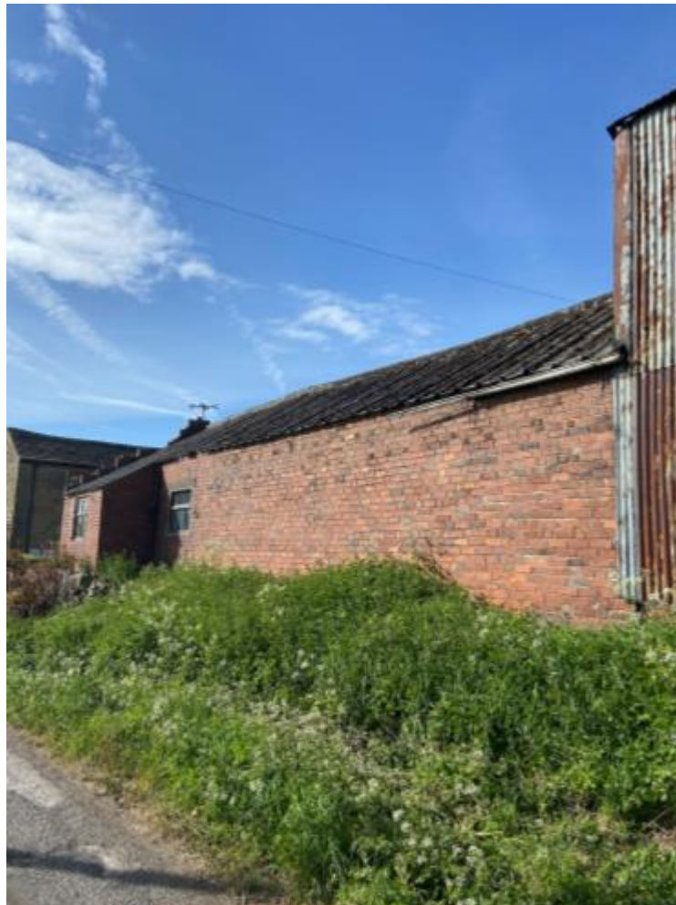
Photo P1A – Pony Stable Walls to Hunshelf Road Elevation
