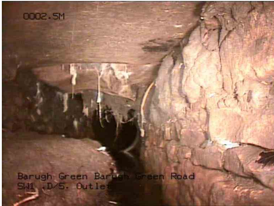
1, 00:00:54, 2.50 m Settled deposits, other, 30% cross-sectional area loss, Mud
