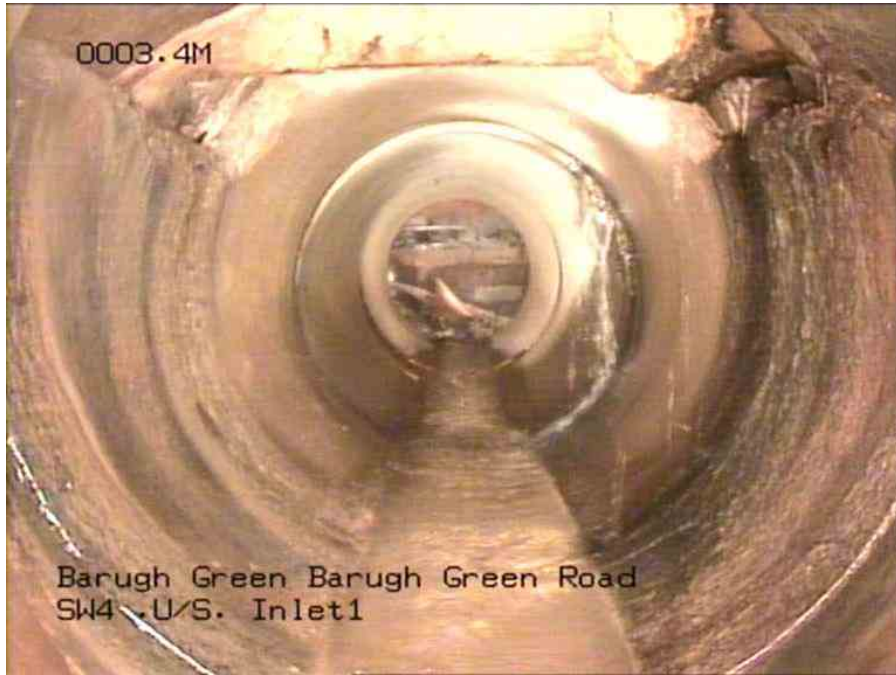
1, 00:00:47, 3.40 m Other obstacles from 11 o'clock to 1 o'clock, 5% cross-sectional area loss, Service Pipe
