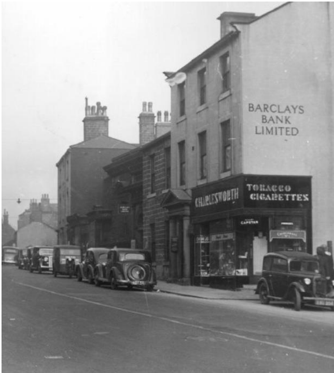
Fig 02. Archive photograph of 23 Church Street (taken from the south-west) (c. 1930).
