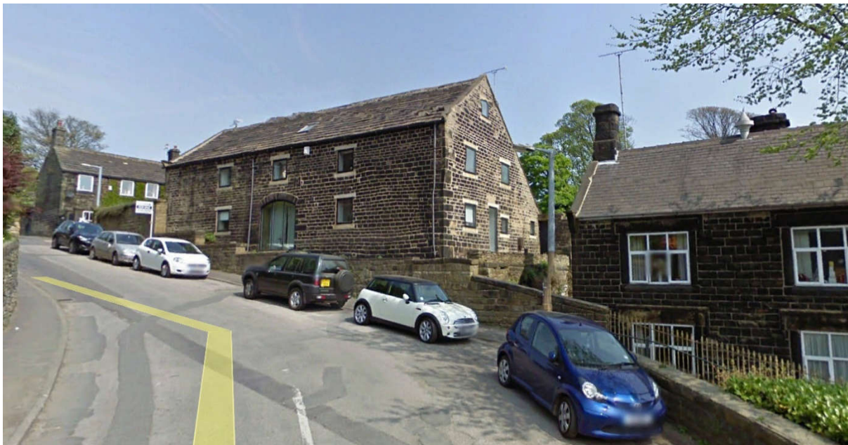
Fig 12. Towngate looking north east towards Redminster Barn.
