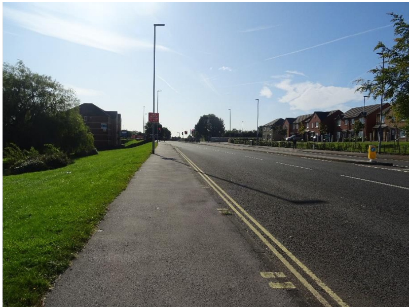
Photo 1: Footway on Broadway
