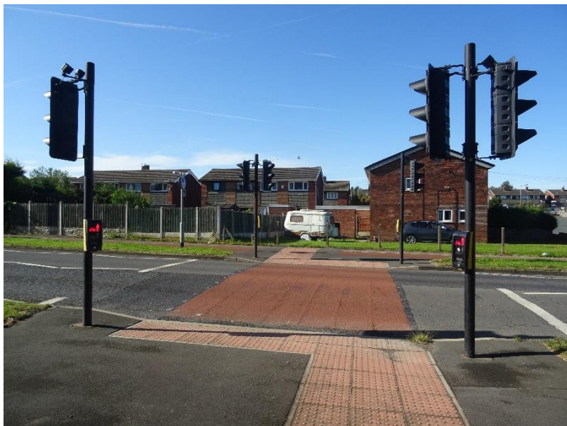
Photo 3: Toucan Crossing on Broadway
