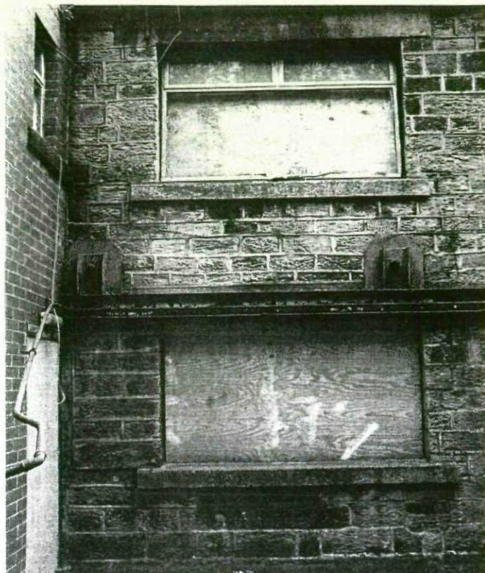
Plate 7 Rear elevation showing strapping directly above ground floor window opening, with brackets attached thereto which form bearing plates for tie bars
