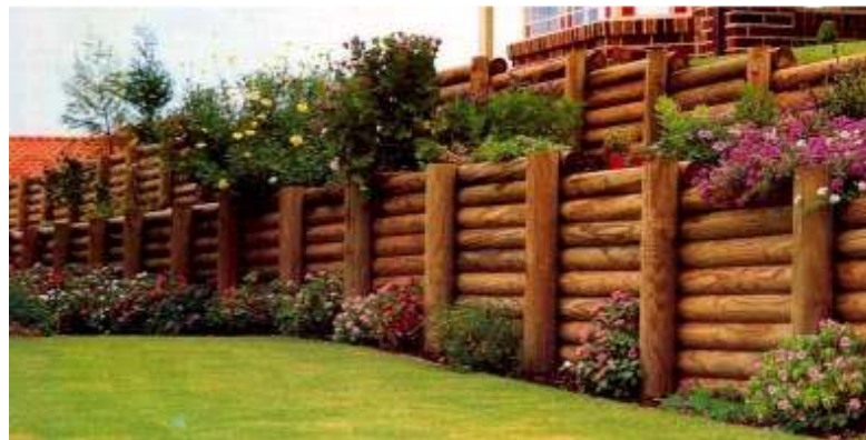
Timber log retaining wall
