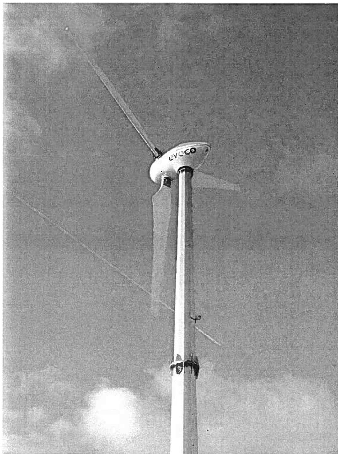
THIS IMAGE SHOWS THE CLEAN DESIGN OF THE EVOCO 10 AND WITH THE WHITE COMPOSITE BLADES, WHITE NACELLE BODY AND GALVANISED STEEL TOWER.
