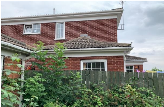
Windows to the side of number 8 facing the applicant's property.
