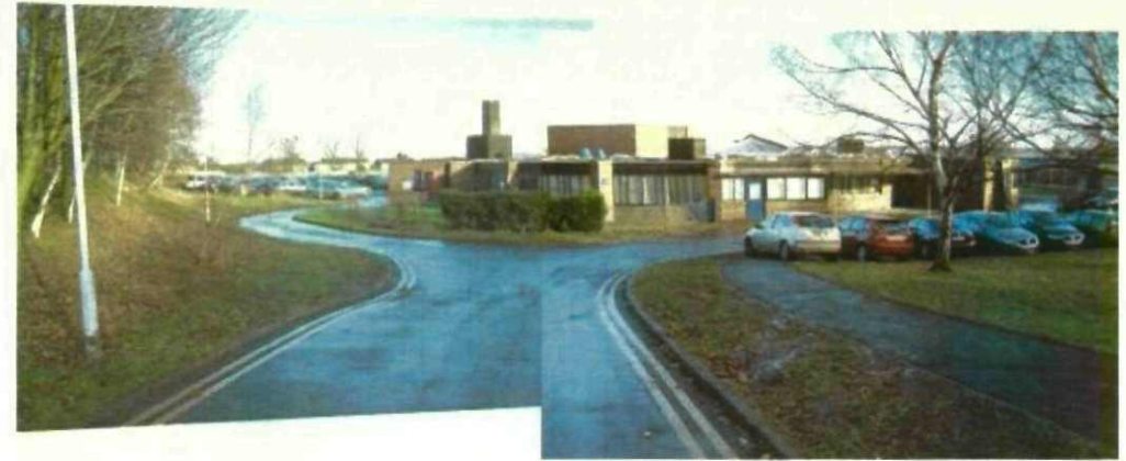
Fig. 4 The existing building viewed from the main entrance looking North
