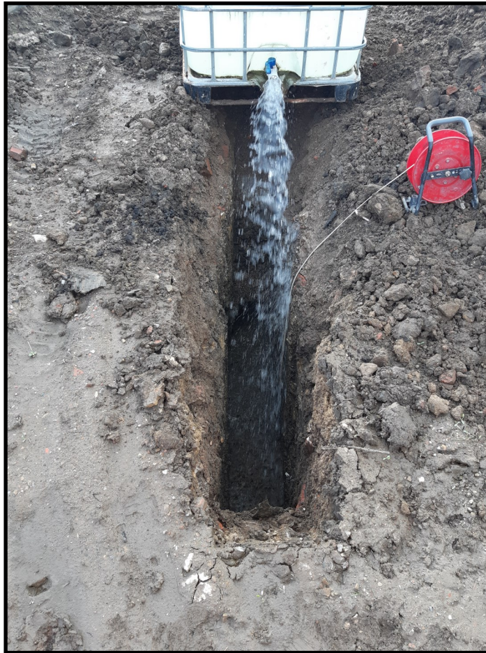
Photograph 21: TP05 soakaway test
