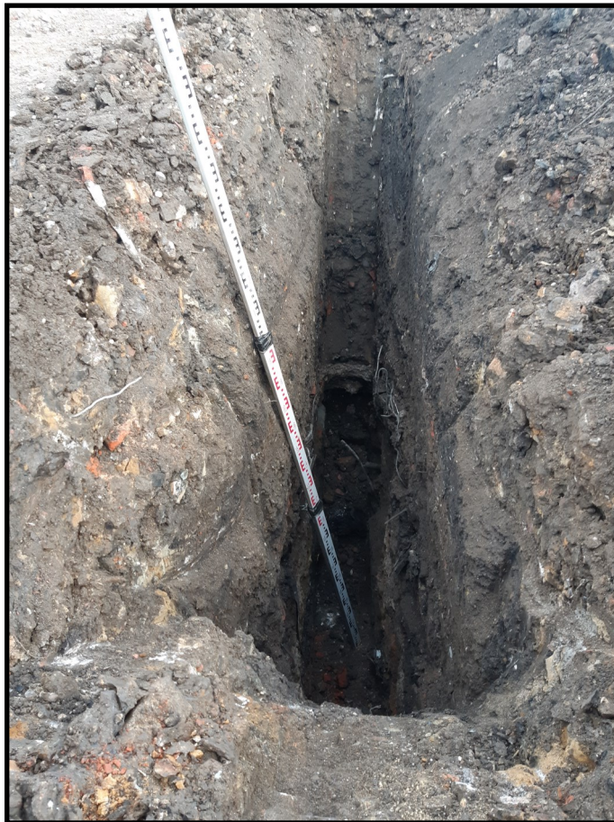
Photograph 25: TP07, base at 2.8m bgl
