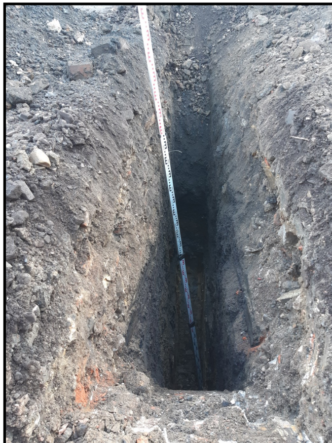
Photograph 16: TP02, base at 3.5m bgl.
