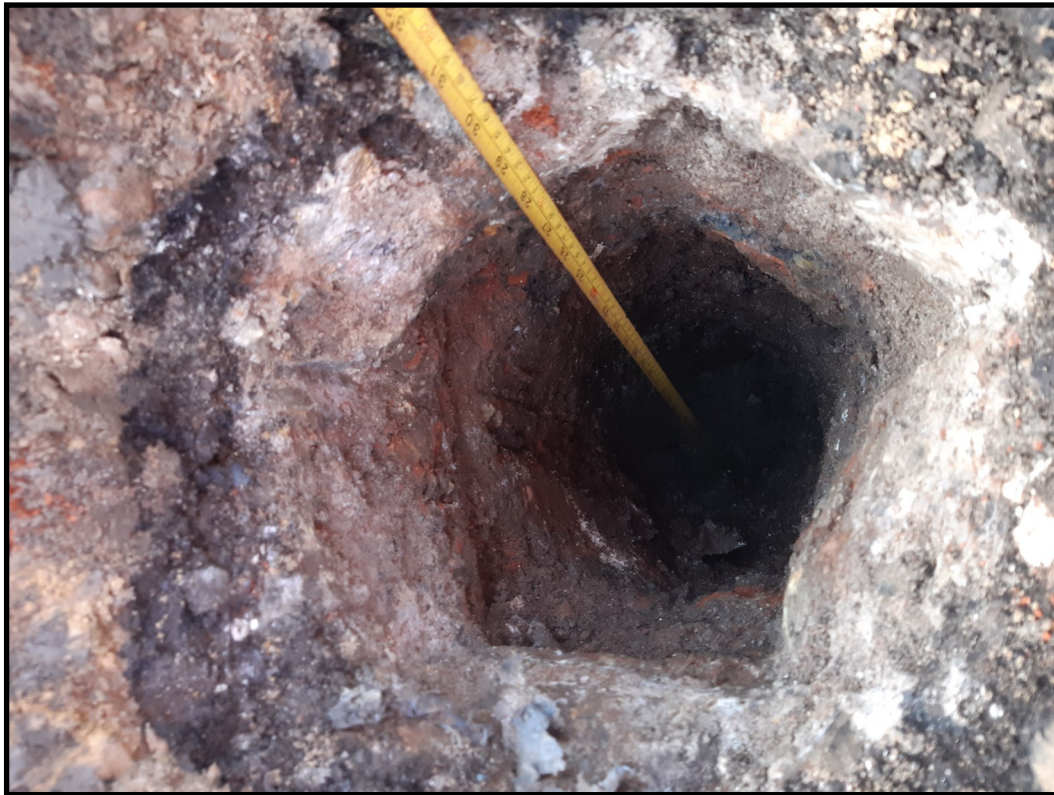
Photograph 1: WS01 Inspection pit
