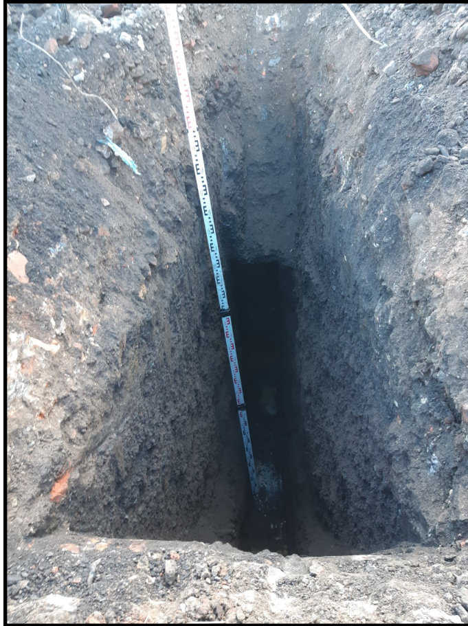
Photograph 13: TP01, base 3.4m bgl.
