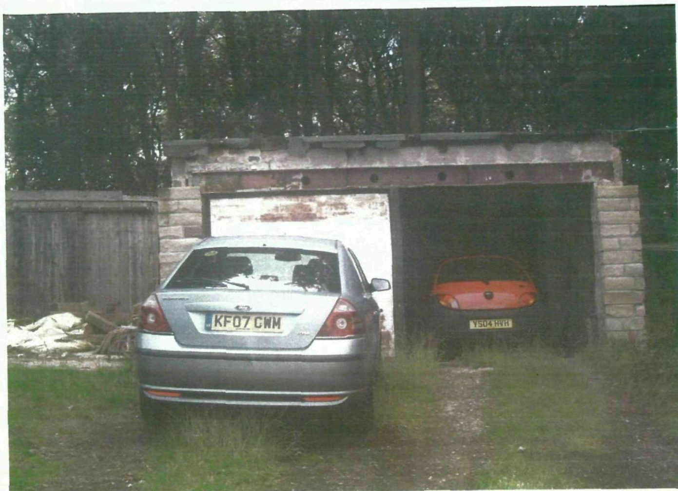
EXISTING GARAGE, THE PARSENAGE, BROOKHILL LANE, CARLETON
