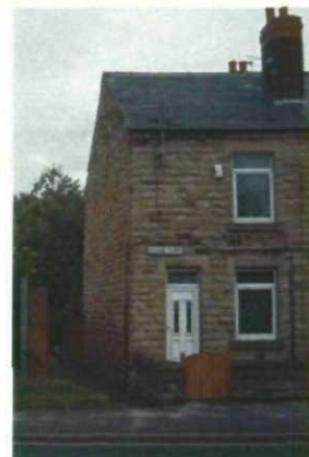
Terraced properties in stone and brick with slate roofs
