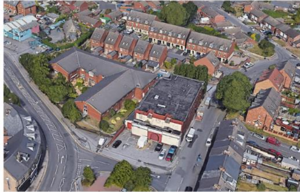
Existing 2024 google map aerial image. The large rectangular design of the old cinema building no longer fits amongst its residential surroundings and sits tight to the street.
