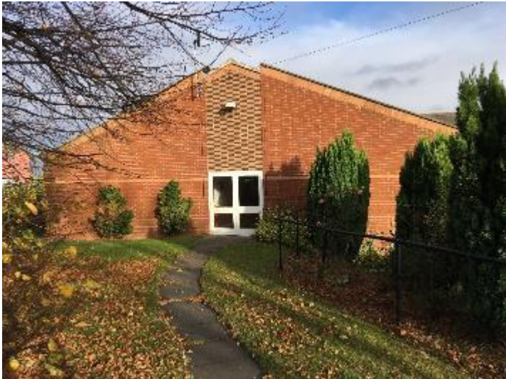
A wing of the care home facing Barnsley Road
