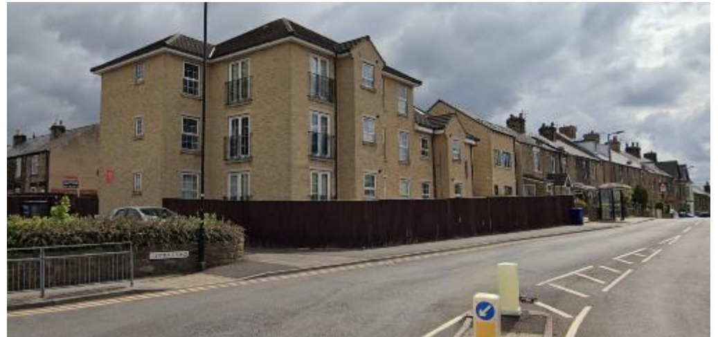
New row Court Flats seen from Barnsley Road and no more than 75 metres from the Care Home are 3 Storey and of simple design
