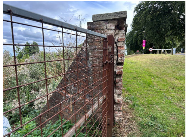
Brickwork and steel column post to the right hand side where the gate opening has been widened
