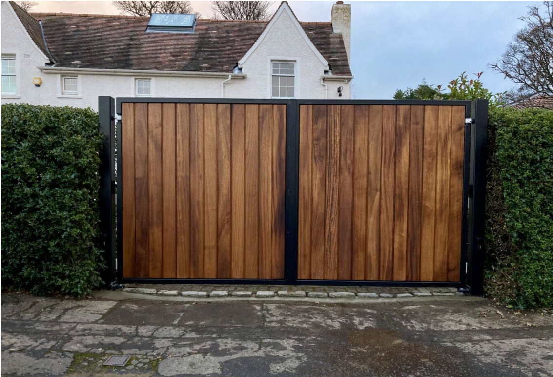
Figure 4: Example image of similar gate design with steel frame and vertical timber infill panels
