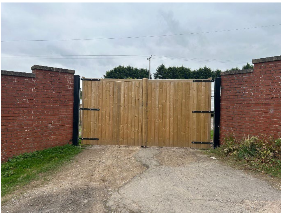
Figure 5: Existing North Gate Entrance
