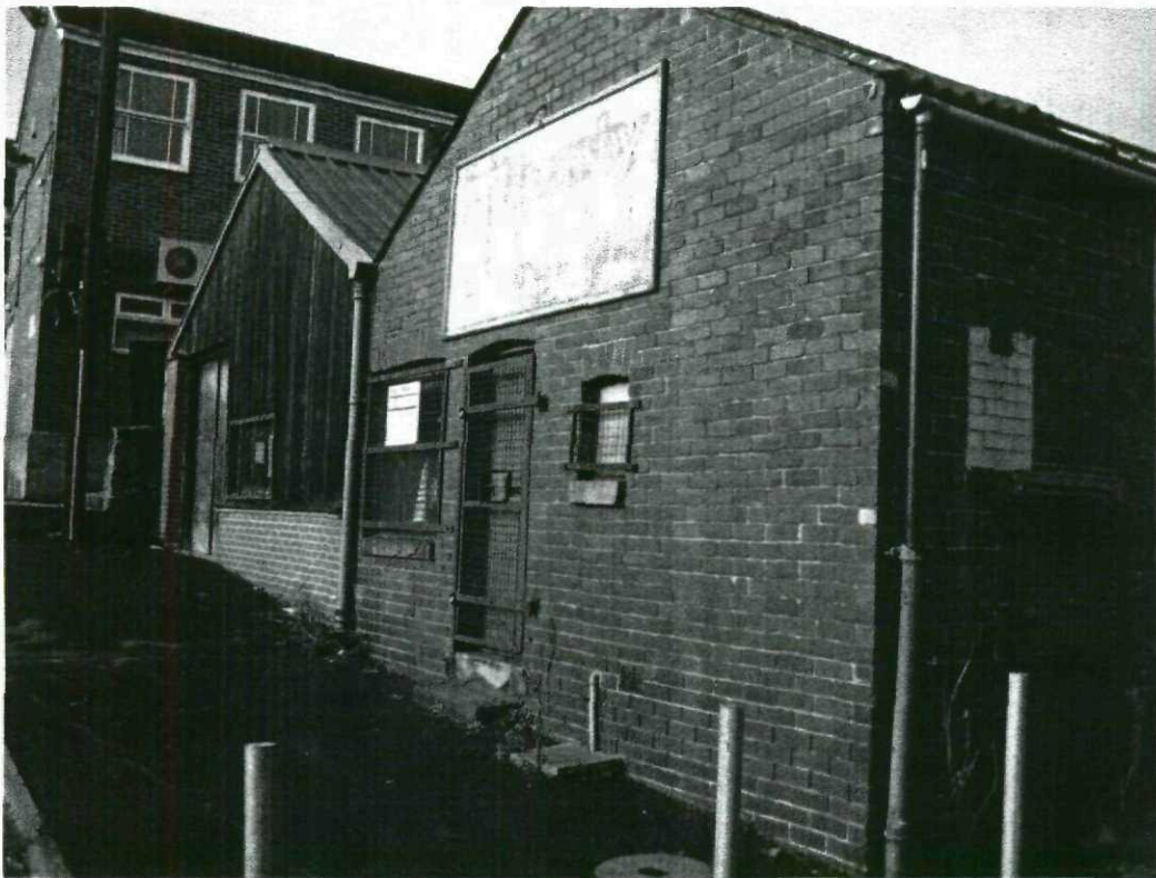
Photograph 6 Front elevation of on site building with Locky's fitness studio extension in the background.
