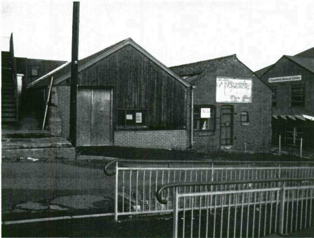
Photograph 7 front elevation of on site building to be demolished, with a partial view of Chapelfield medical centre shown to the right
