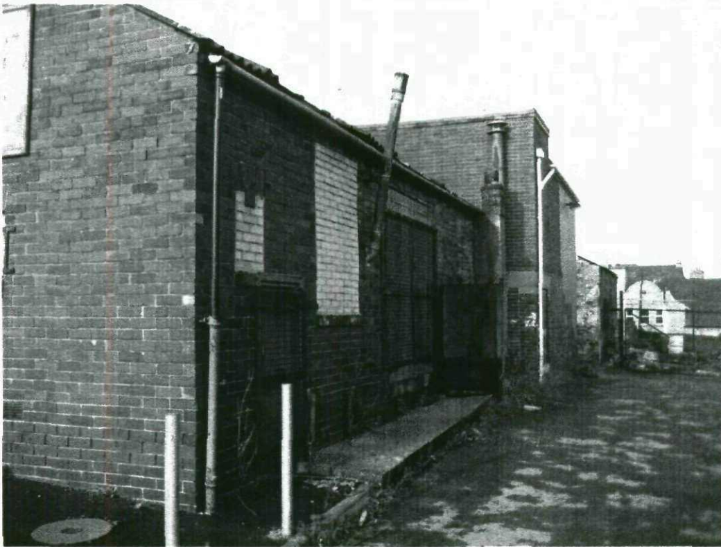
Photograph 5 View showing elevation of existing building abutting link road in the foreground and Locky's building in the background.
