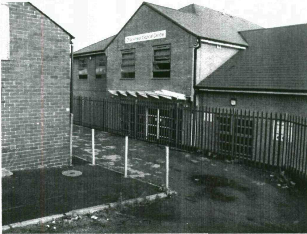
Photograph 3 Intersection of link road connecting AR1 to AR2 running between Chapelfield Medical Centre and the existing site building.
