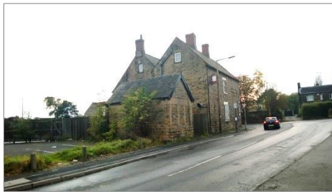
Wharncliffe Arms, Carlton, Barnsley
