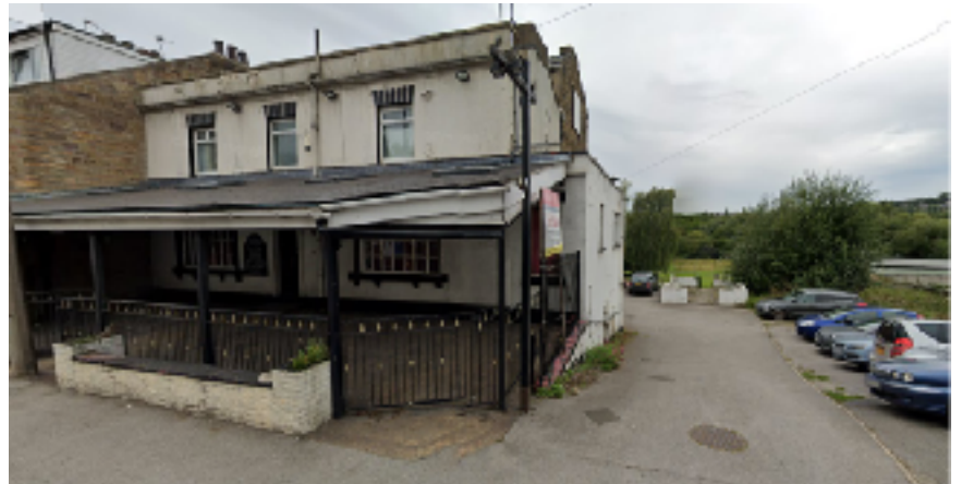
Image 1 – Existing view of the application site looking north from Pontefract Road.
