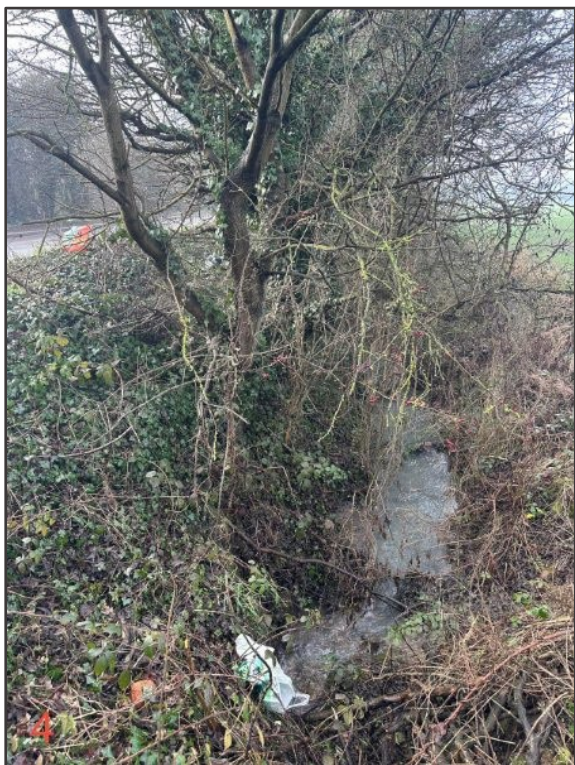
Picture 3. G4#. Ditch with flowing water
