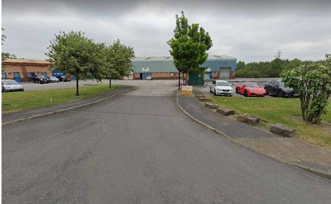
Photo 1 – Site Access of Stairfoot BESS
