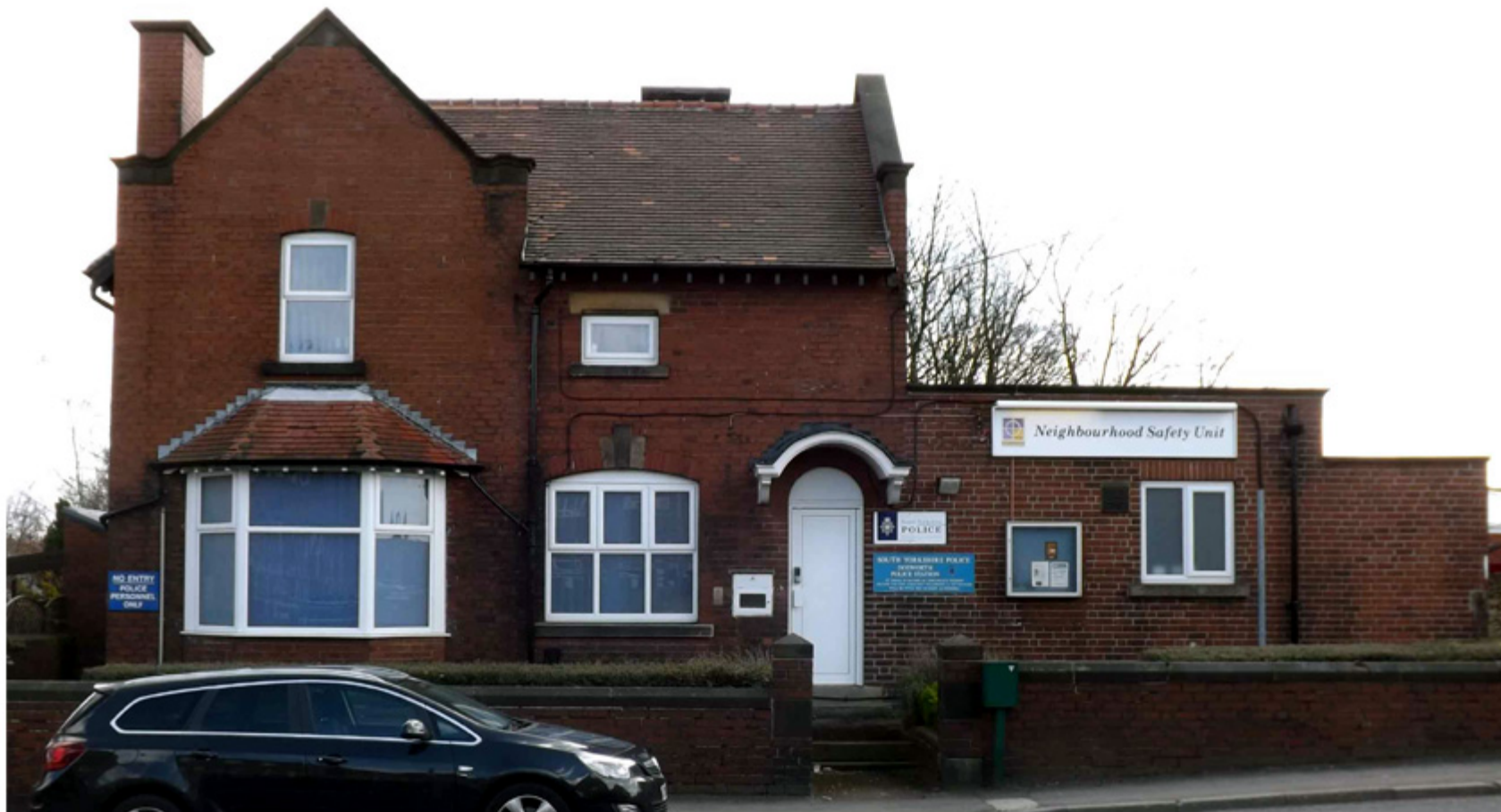
Dodworth Police Station: As Existing
