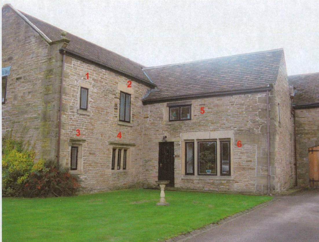
Picture 1 Front (east) elevation (a)
