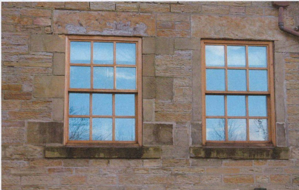
Picture 4 Double hung oak sash
