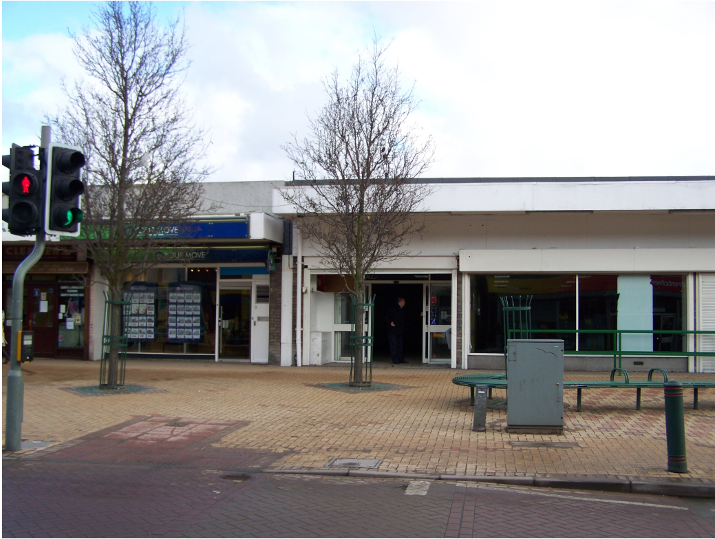
Photo 1: Existing High Street shop front entrance.
