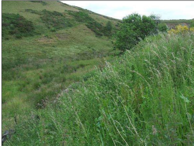
Photo 4: Current Site Condition – View north east along the top of the embankment extending along the north eastern edge of the site.
