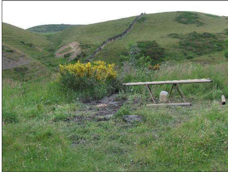
Photo 13: RBH02 – Borehole location upon completion showing cover to gas monitoring well installation (light brown area near gorse bush).
