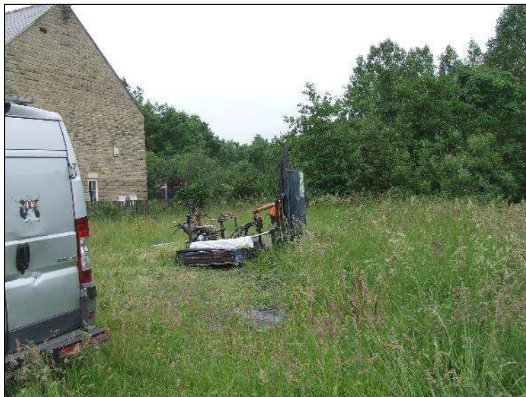
Photo 2: Current Site Condition – View of north western end of site looking west (window sampling rig is set up on WS03).
