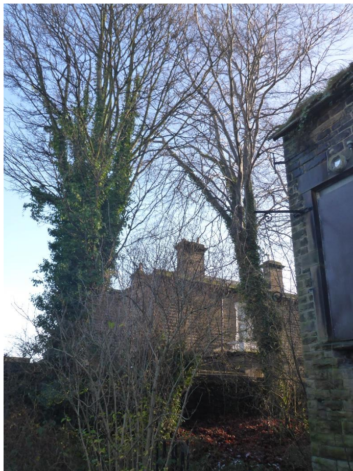
Photo 2: T2 and T3 (left to right) situated close to the existing building.
