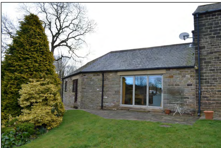
Figure 11: View of the west elevation of the north extension, looking north-east
