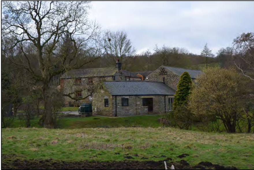
Figure 6: View of Ash Barn from Finkle Street Lane, looking south.
