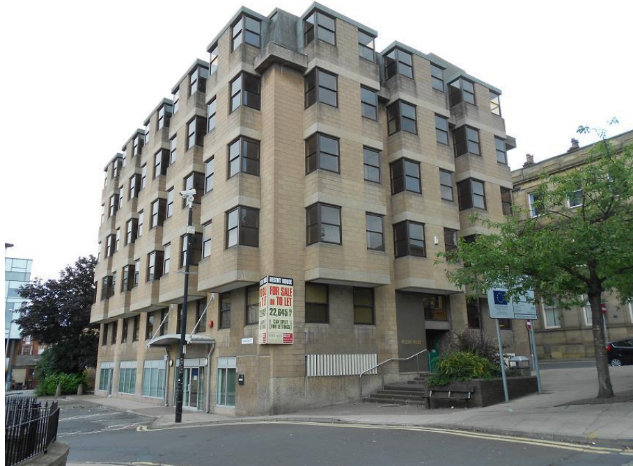
View of Regent House from Regent Street
