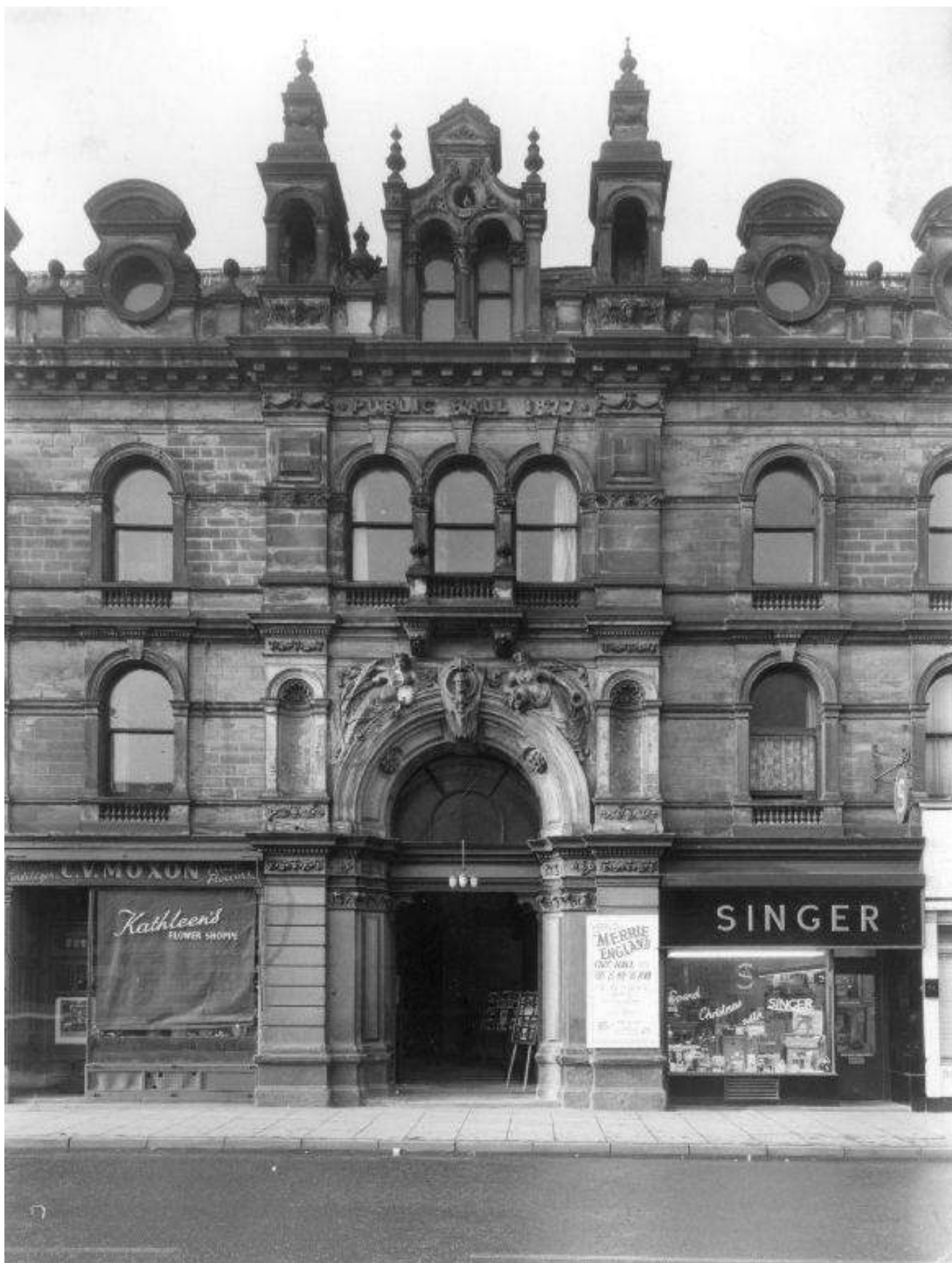
Fig. 24: Archive Image of Entrance 1963
