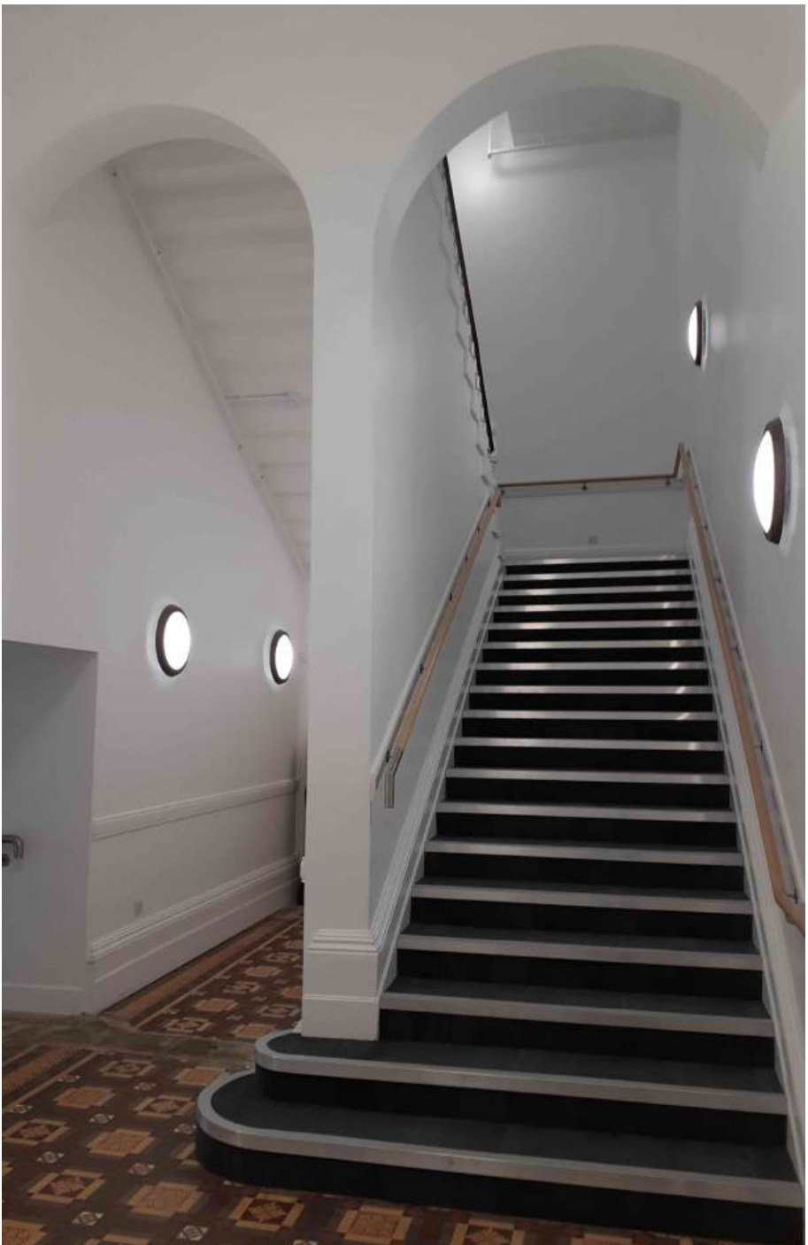
Main stairwell (south) - stair behind partition with original encaustic floor tiles visible.
