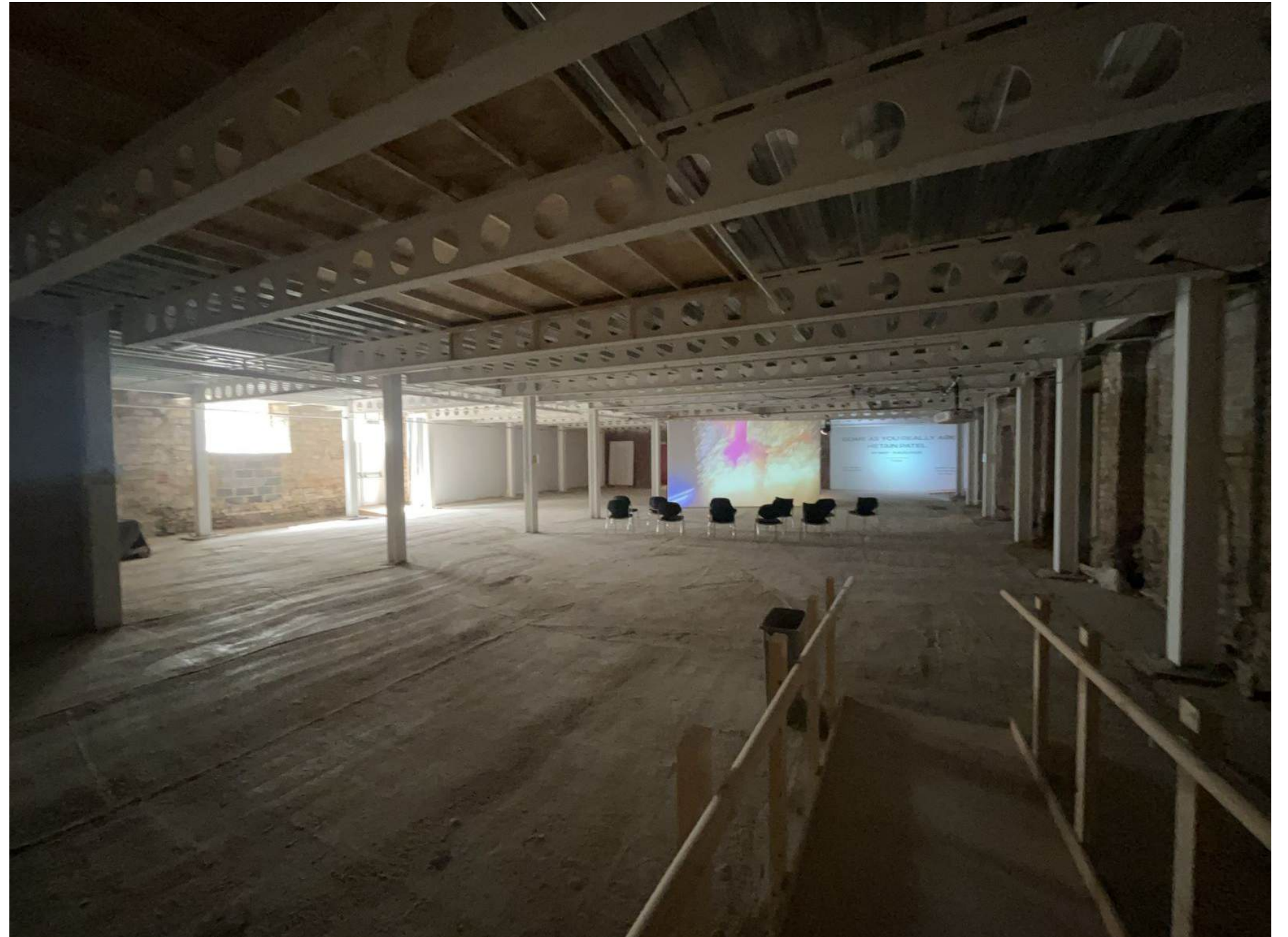
Ground floor hall space looking west with temporary event. Internal side of south elevation visible including window, external door and wall lining concealing infilled and vented openings.
