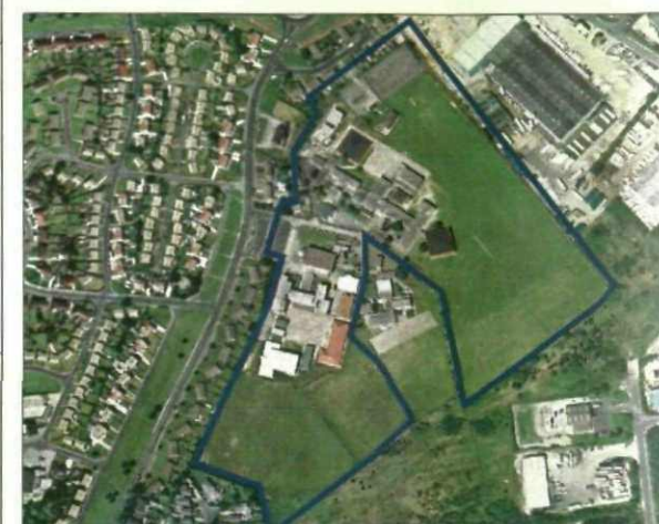
AERIAL VIEW OF EXISTING SITE
