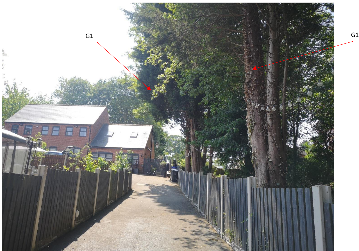
Photo 10: looking north down existing tarmac driveway
