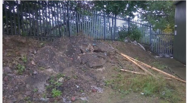
North-East boundary note showing steep incline to surrounding ground level
