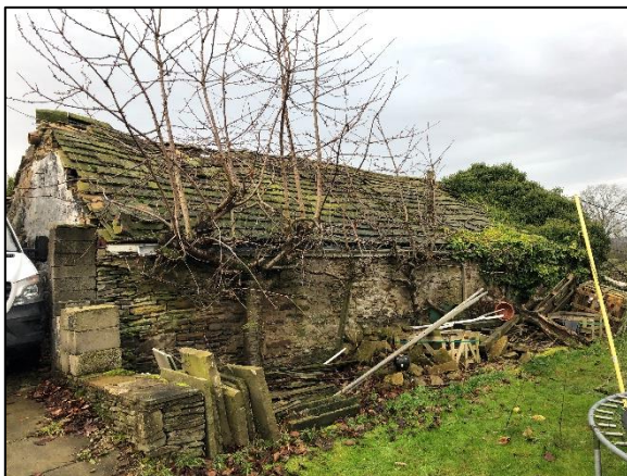
Figure 3: The northern elevation of the building.
