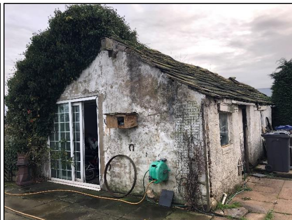
Figure 4: The western elevation of the building.
