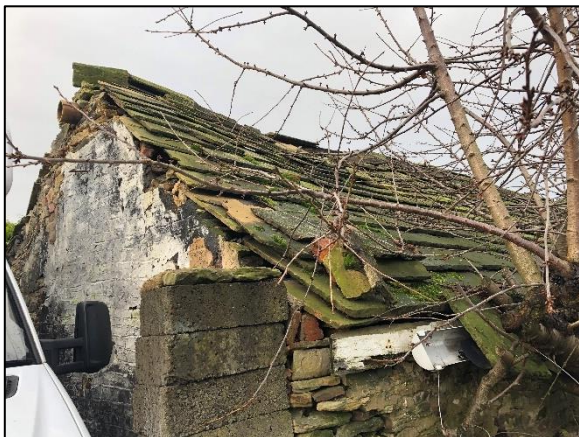
Figure 8: The eastern elevation of the building.
