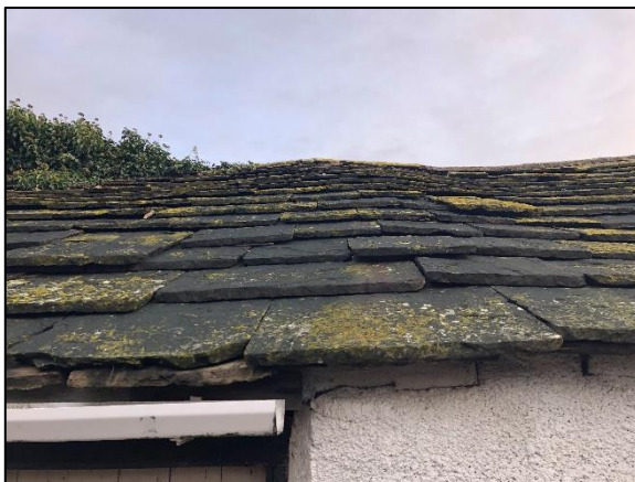
Figure 11: The stone tiles on the roof of the building.
