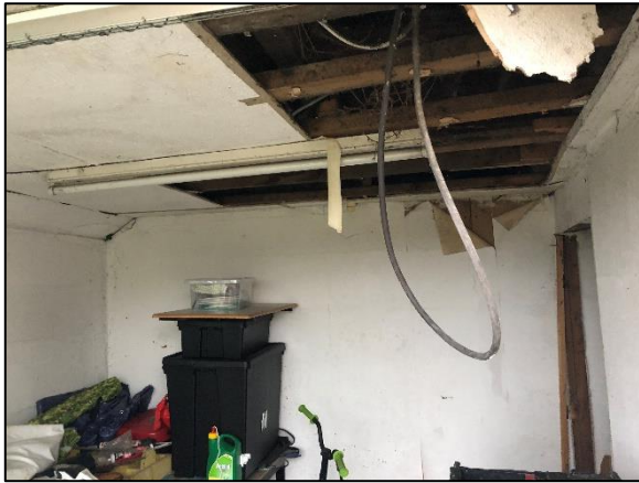
Figure 5: The interior of the western end of the building.
