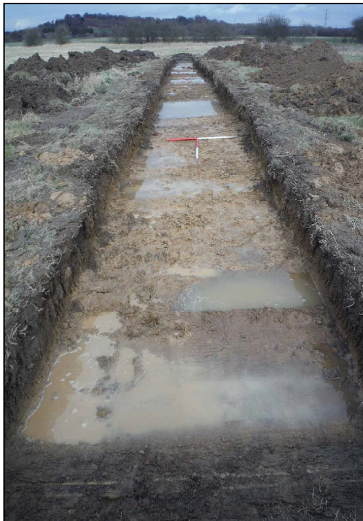
Plate 12. Trench 15, lookng north-east
